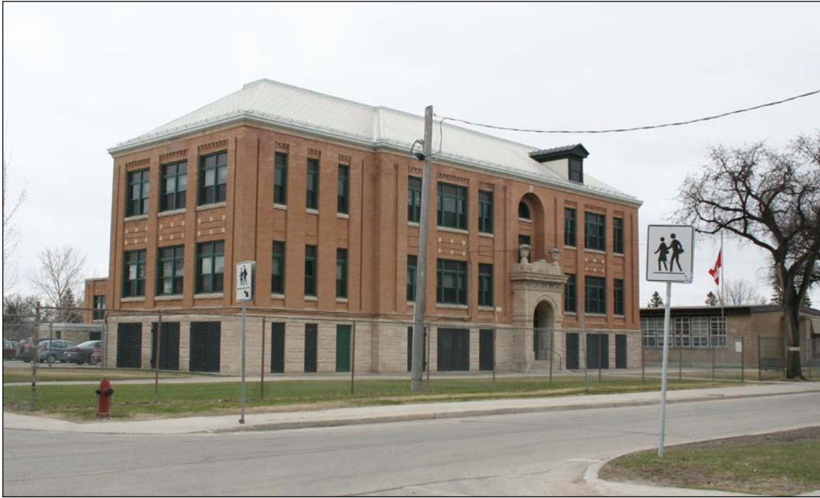
North and west façades, 2009
