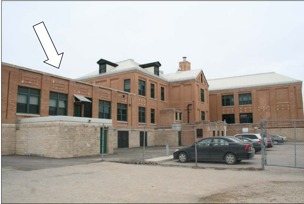
Rear of school including 1948 addition (arrow), 2009
