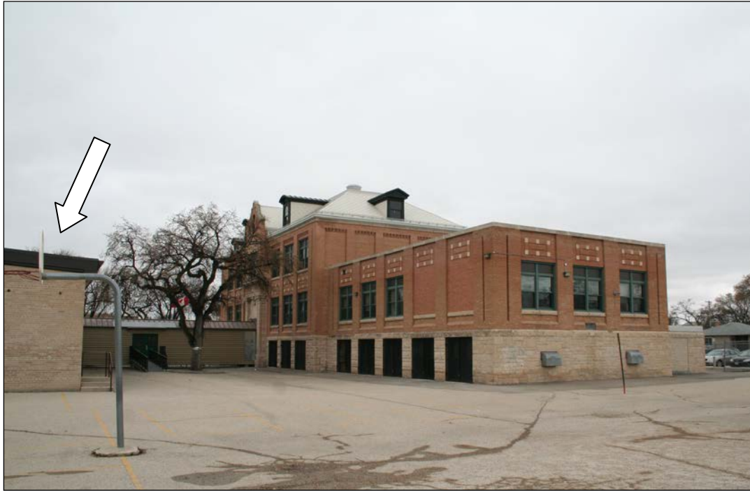
South and east façades and one-storey addition (arrow), 2009
