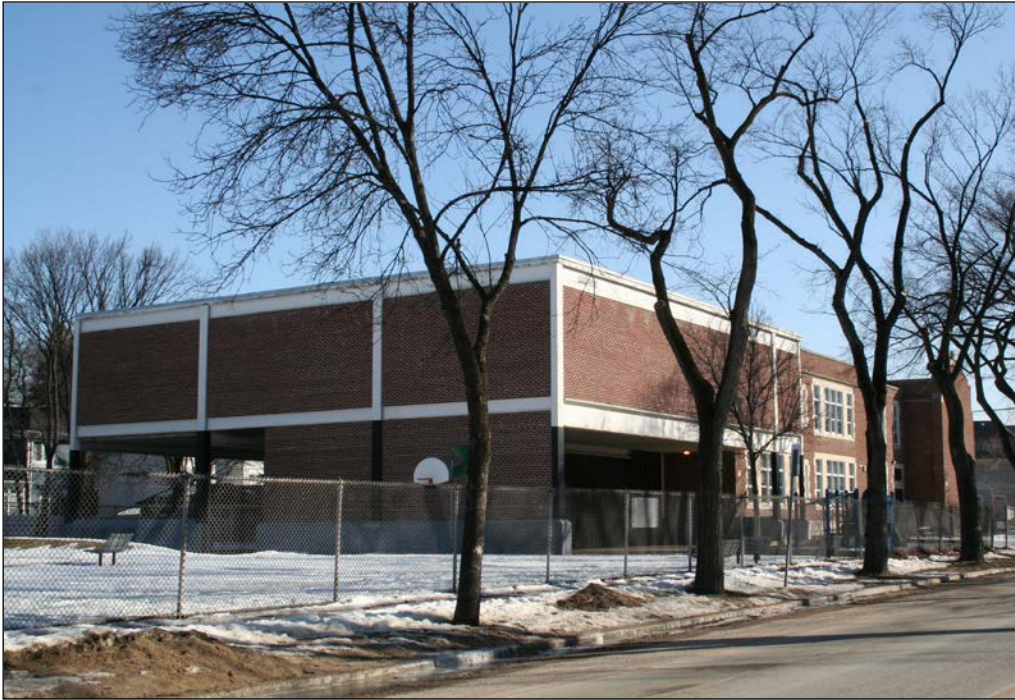
West and south façades, 2009
