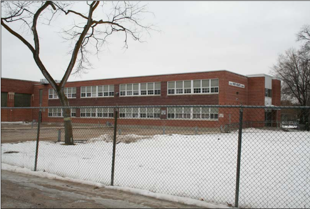
Rear (east) and north façades, 2008
