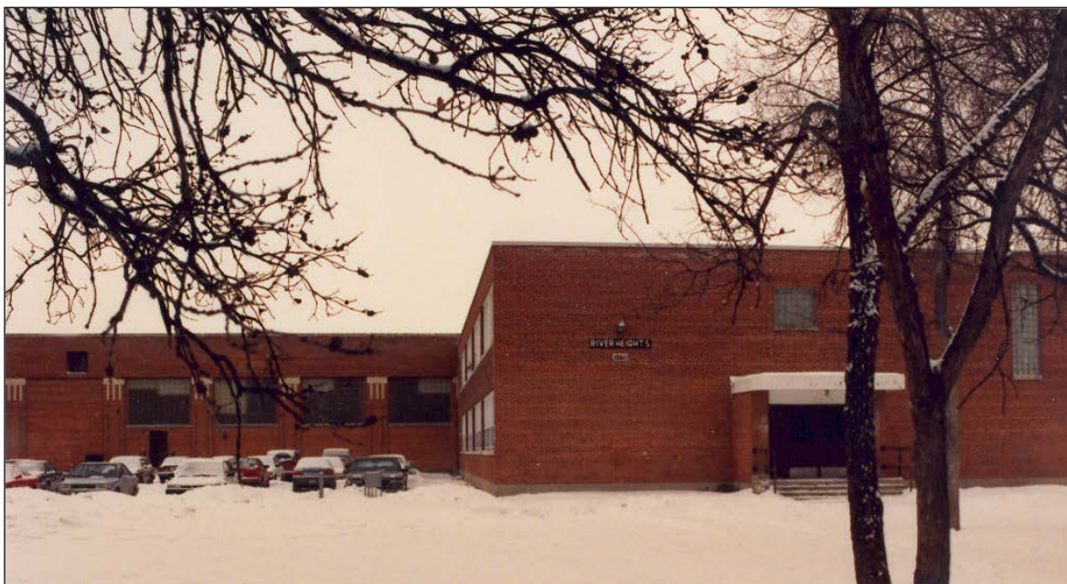
North façade, no date
