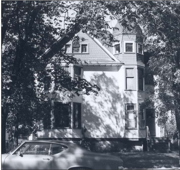
Front (south) façade, 1978
