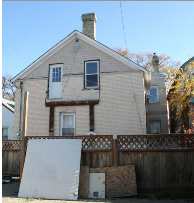
Rear (north) and west façades, 2007
