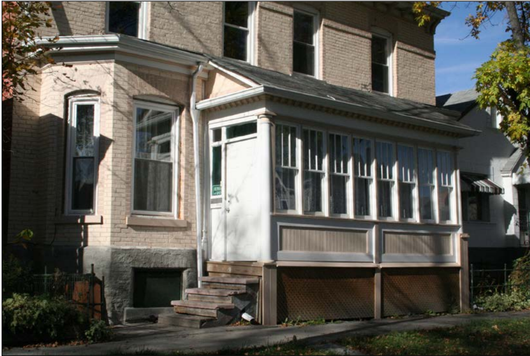
Detail of front (south) façade, 2007
