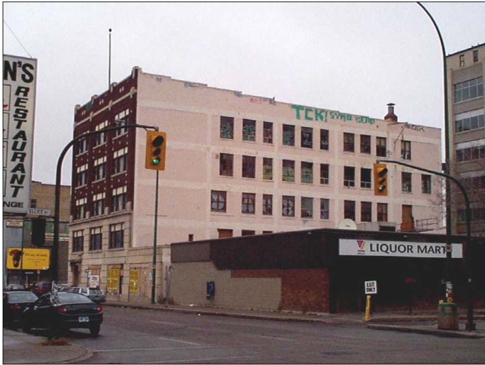
Plate 8 – South façade. ( M. Peterson, 2001. )
