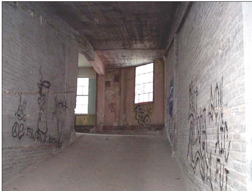
Plate 11 – Vehicle ramp to second floor. ( M. Peterson, 2001. )
