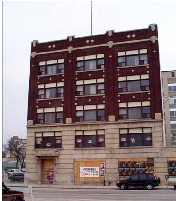
Plate 2 – Front (west) façade. ( M. Peterson, 2001. )
