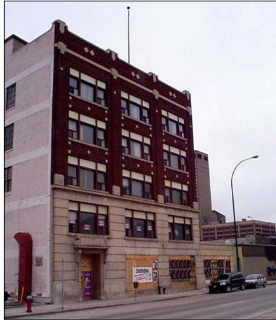
Plate 3 – Front (west) façade. ( M. Peterson, 2001. )
