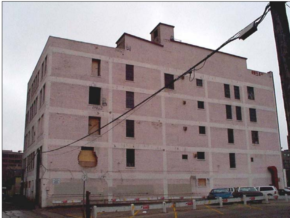
Plate 7 – North façade. ( M. Peterson, 2001. )
