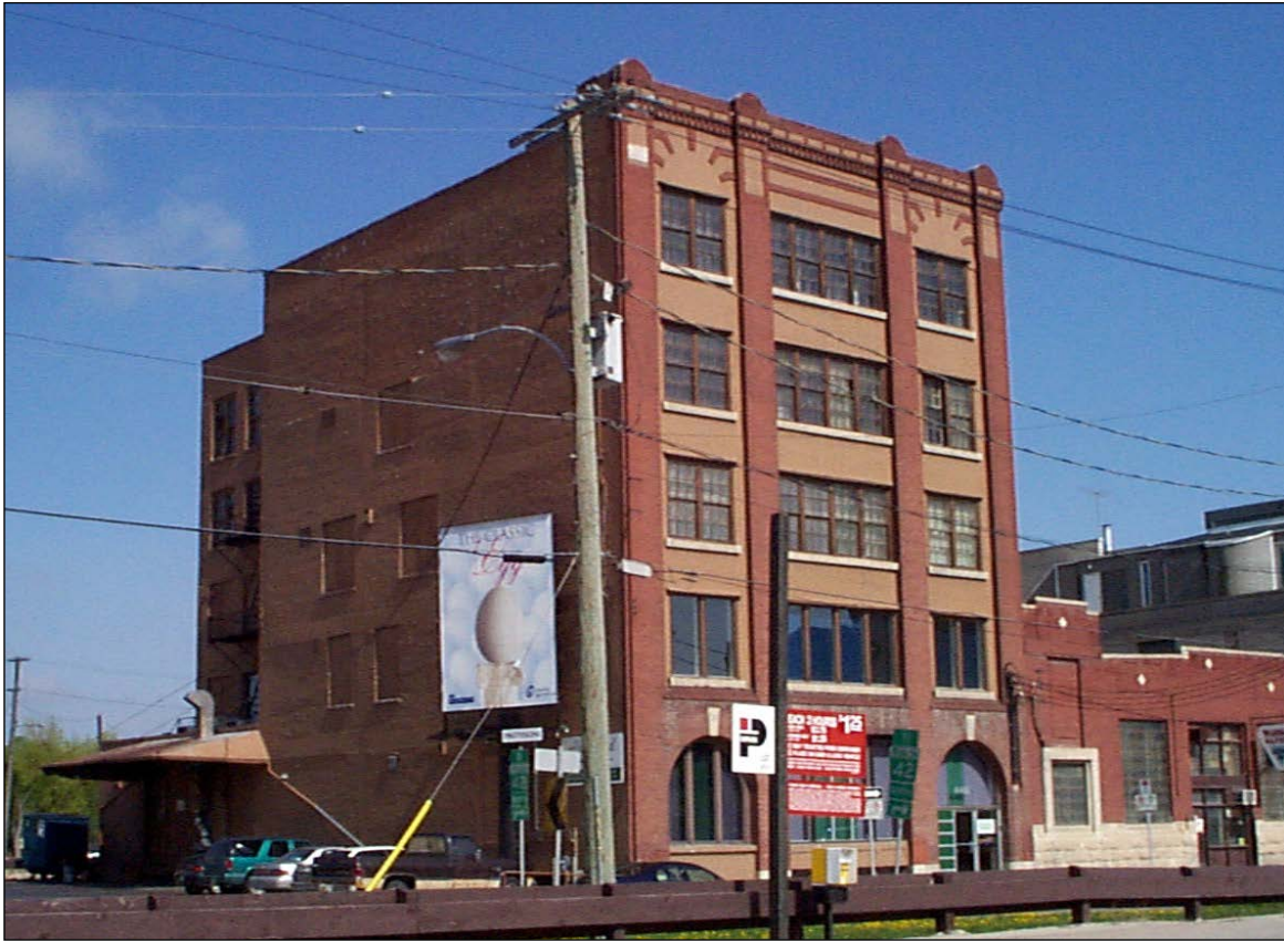
Plate 7 – Clark Brothers Warehouse, 448 Hargrave Street, front (east) and south façades, 1998. ( M. Peterson, 1998. )
