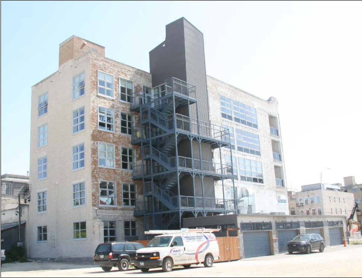
Plate 10 – Clark Brothers Warehouse, 448 Hargrave Street, rear (west) and south façades, 2015. ( M. Peterson, 2015. )
