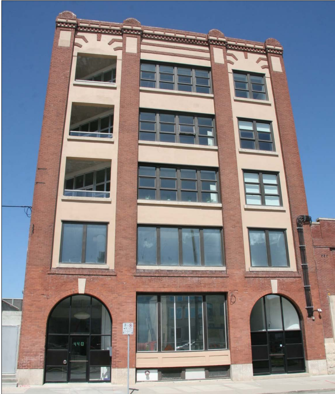
Plate 5 – Clark Brothers Warehouse, 448 Hargrave Street, front (east) façade, 2015. ( M. Peterson, 2015. )
