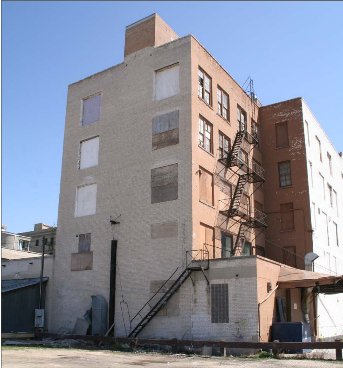
Plate 8 – Clark Brothers Warehouse, 448 Hargrave Street, rear (west) and south façades, 2006. ( M. Peterson, 2006. )
