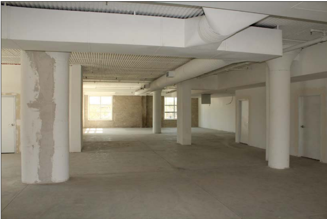
Plate 16 – Clark Brothers Warehouse, 448 Hargrave Street, second floor, 2016. ( M. Peterson, 2016. )
