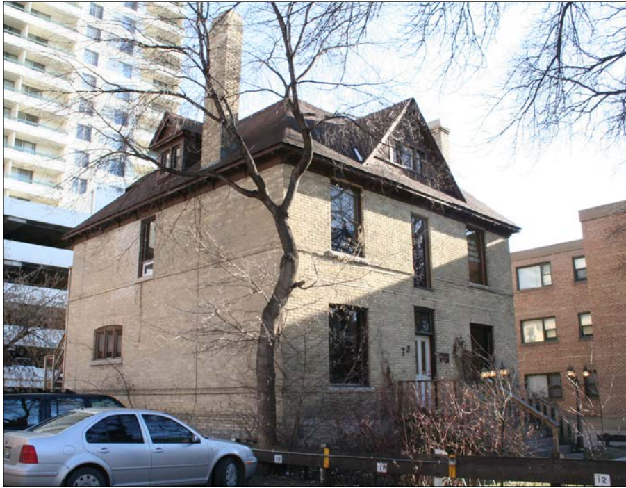
Front (west) and north façades, 2006
