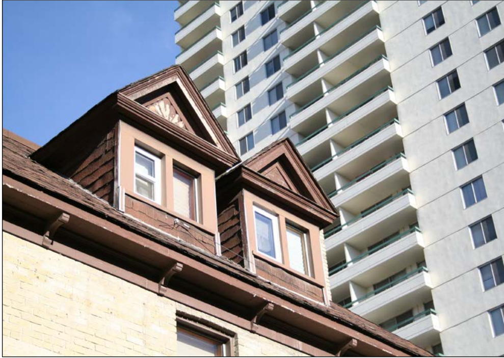
Detail of south side, 2006
