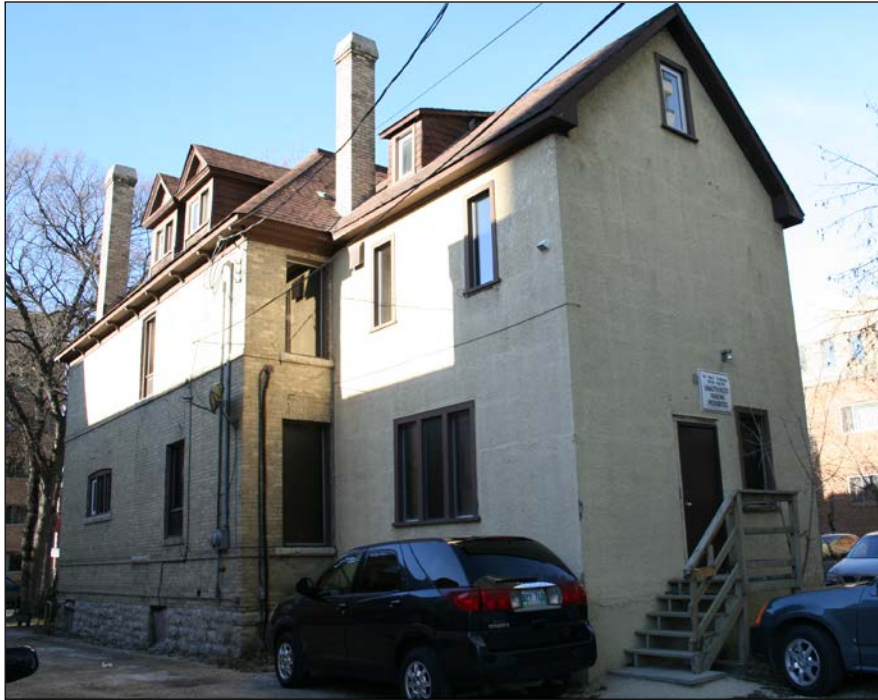
Rear (east) and south façades, 2006
