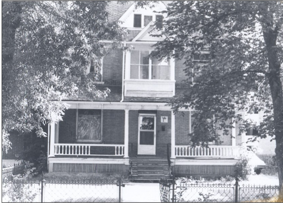
Front (west) façade, 1978, with ornate porch
