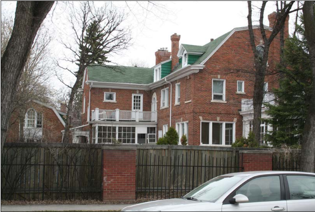
Rear (west) and south façade, 2009
