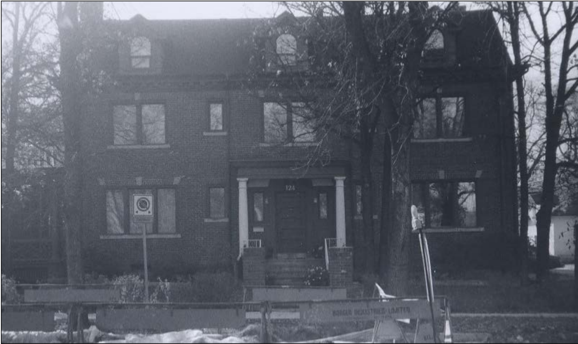
Front (east) façade, 1978
