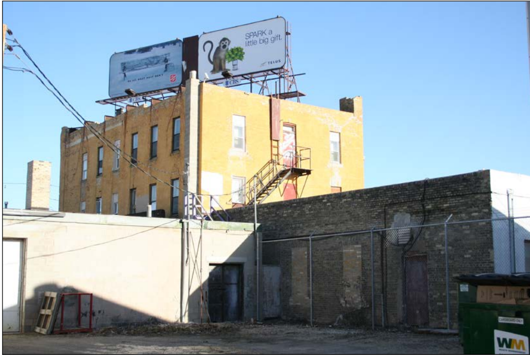
Rear (south) and west façades, 2006
