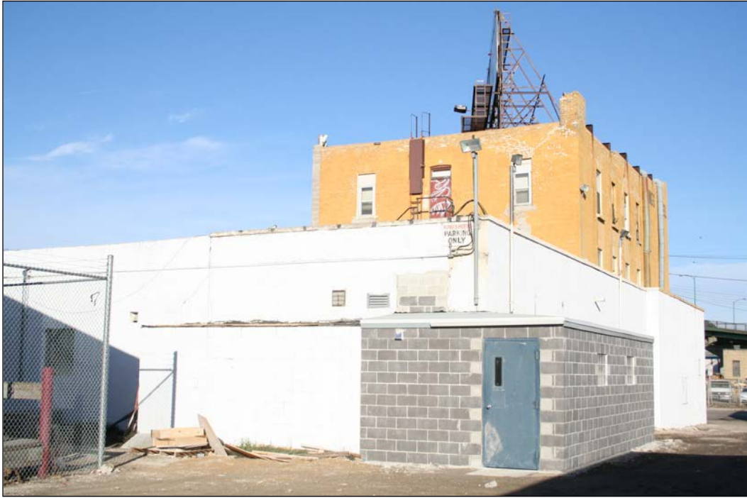
Rear (south) and east façades, 2006
