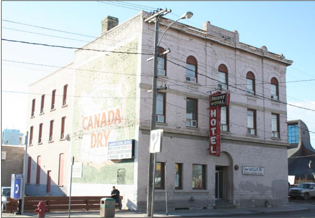
Front (north) and east façades, 2006
