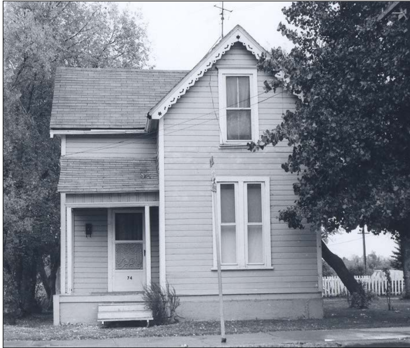
Front (south) façade, 1978
