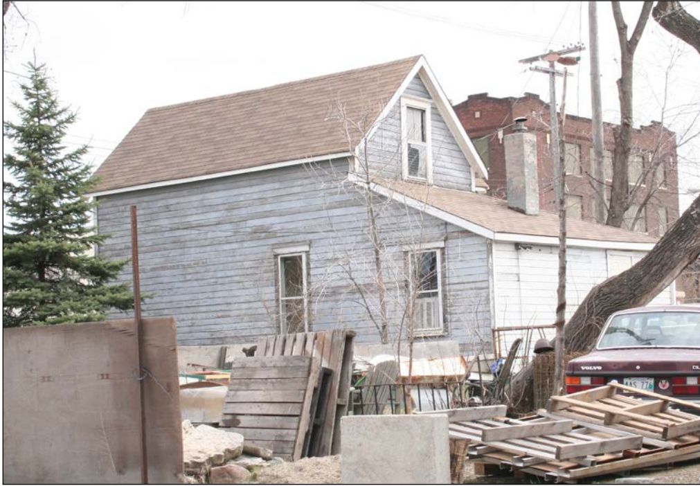
Rear (south) and west façades, 2006
