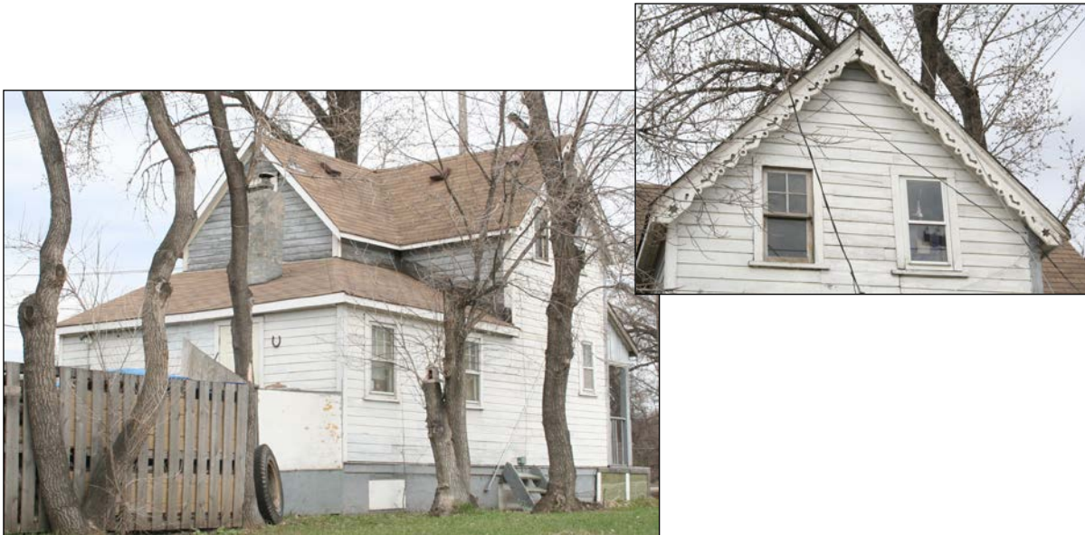
Rear (south) and east façades and detail of east side bargeboard, 2006
