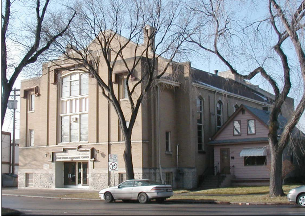
Front (east) and north façades, 2005
