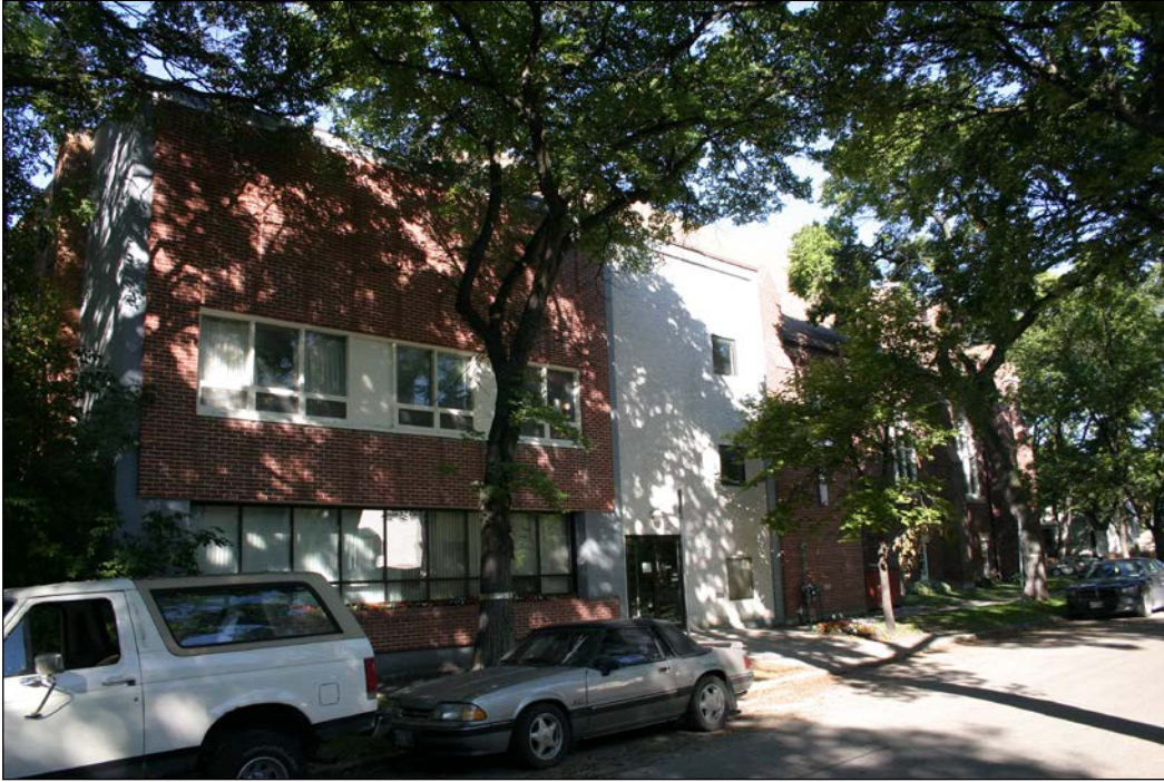
West façade, Christian Education Building, 2009
