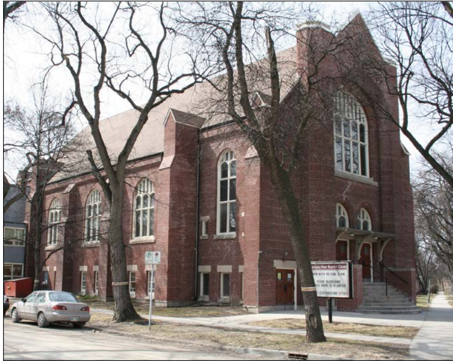
Front (north) and east façades, 2009
