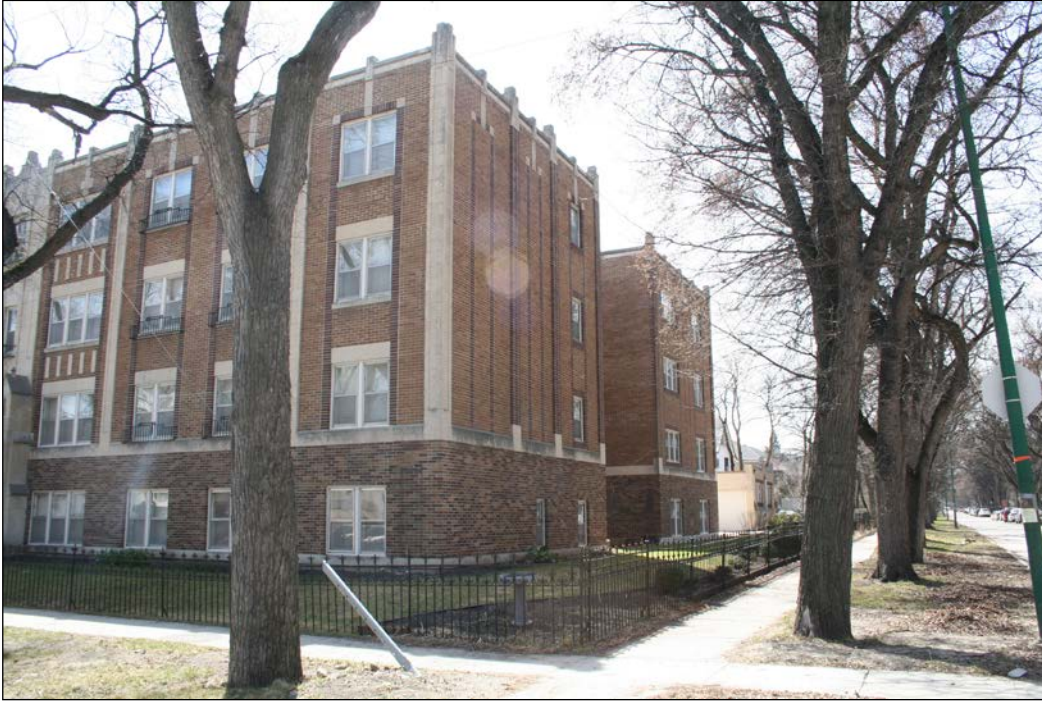
Front (east) and north façades, 2009
