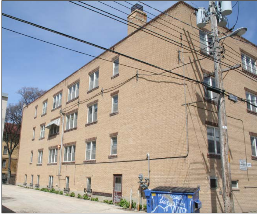
Rear (west) and south façades, 2009
