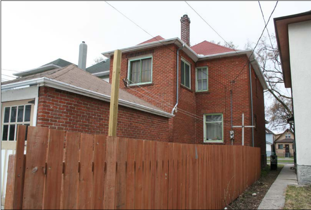
Rear (north) and west façades, 2009
