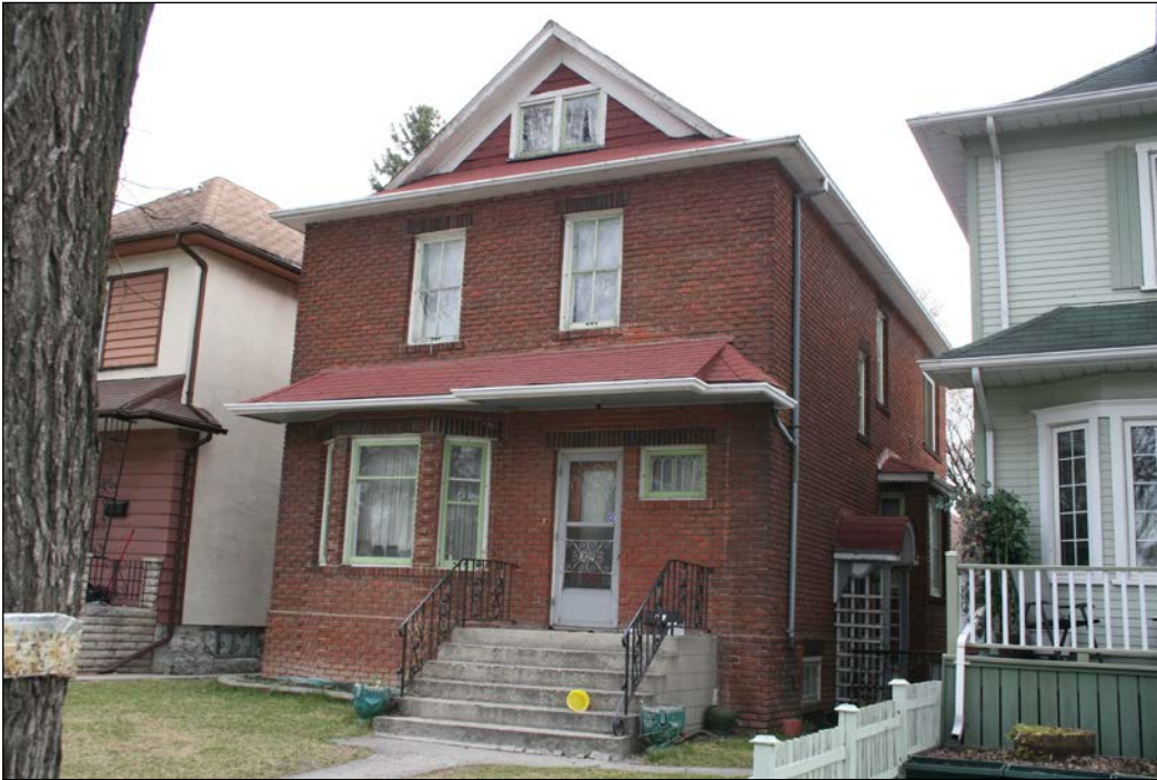
Front (south) and east façades, 2009
