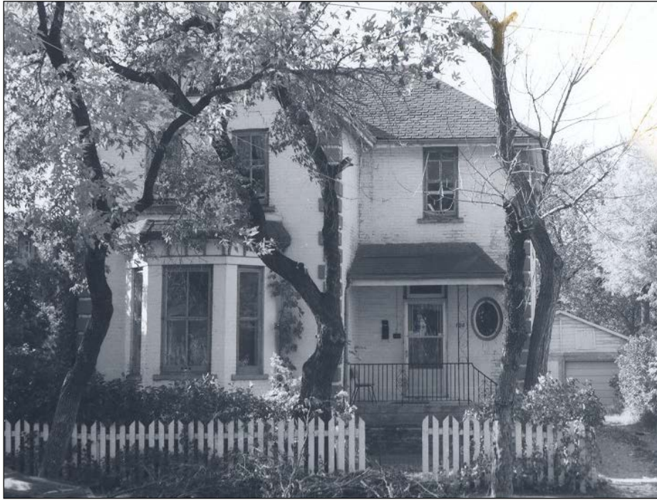
Front (east) façade, 1978
