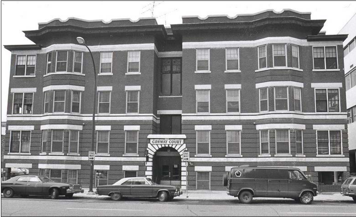
Front (west) façade, 1978
