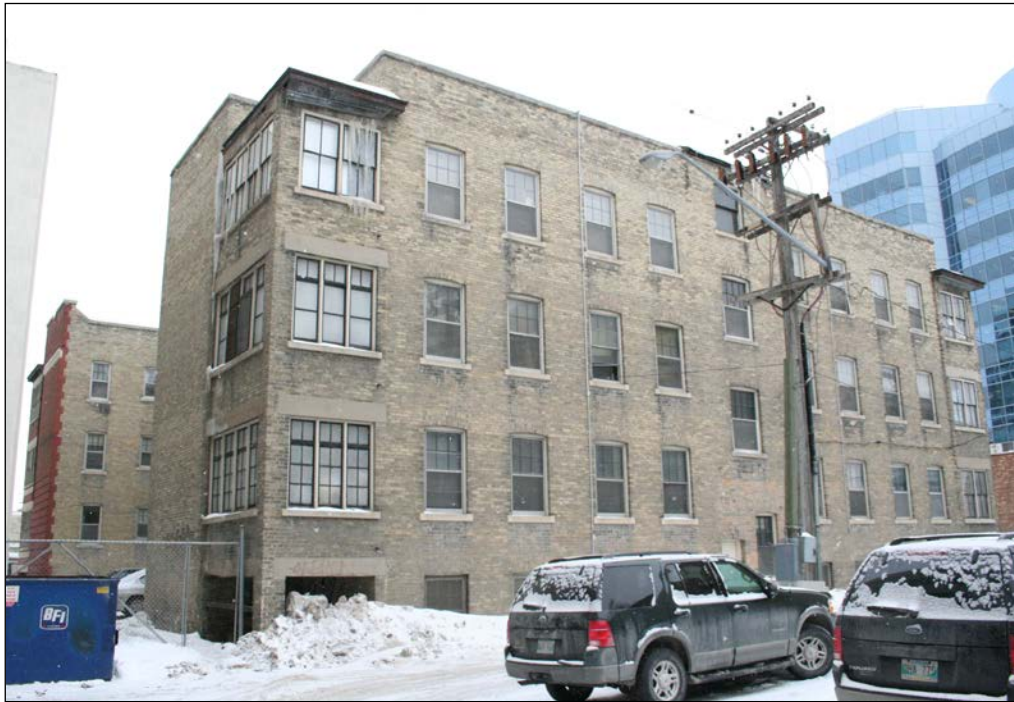
Rear (east) and south façades, 2007
