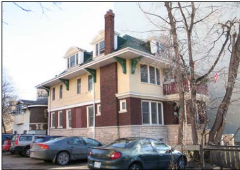
Front (west) and north façades, 2006
