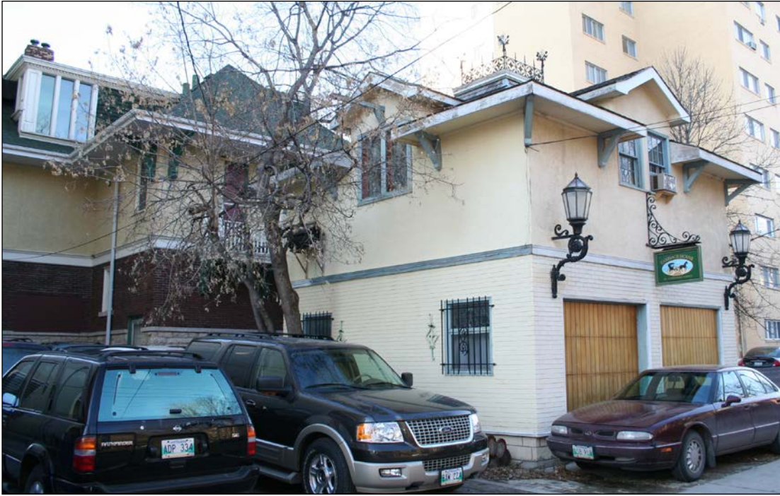
Rear (east) façade of house, east and south facades of the coach house, 2006
