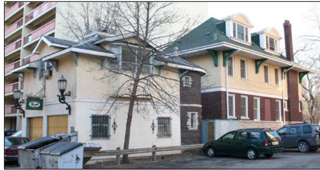
Rear (east) and north façades of house and coach house, 2006
