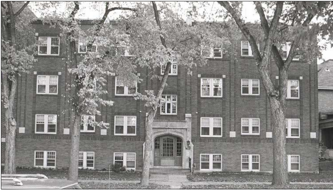
Front (west) façade, 1978
