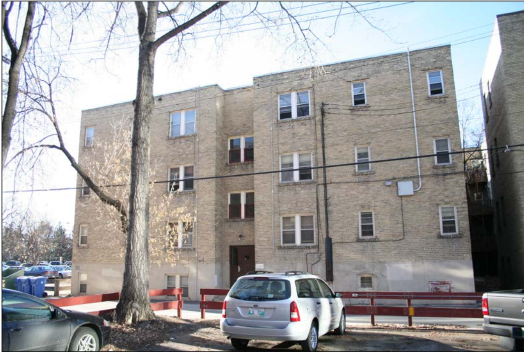
Rear (north) and east façades, 2006
