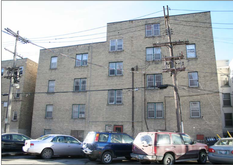
Rear (east) façade, 2006
