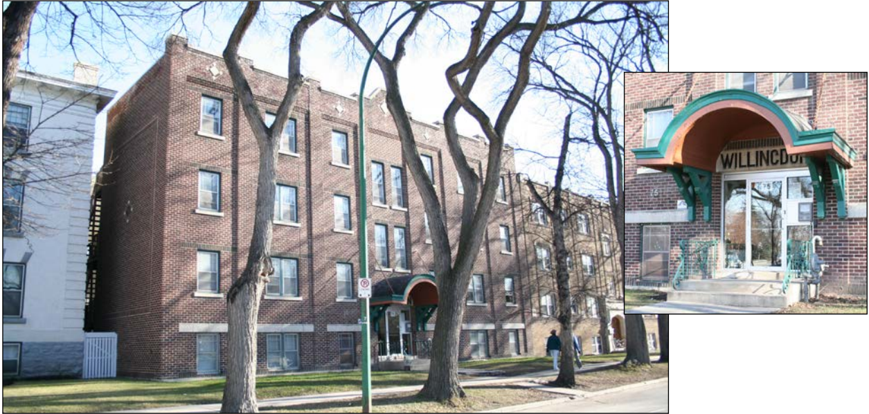
Front (west) and north façades and detail of main entrance, 2006
