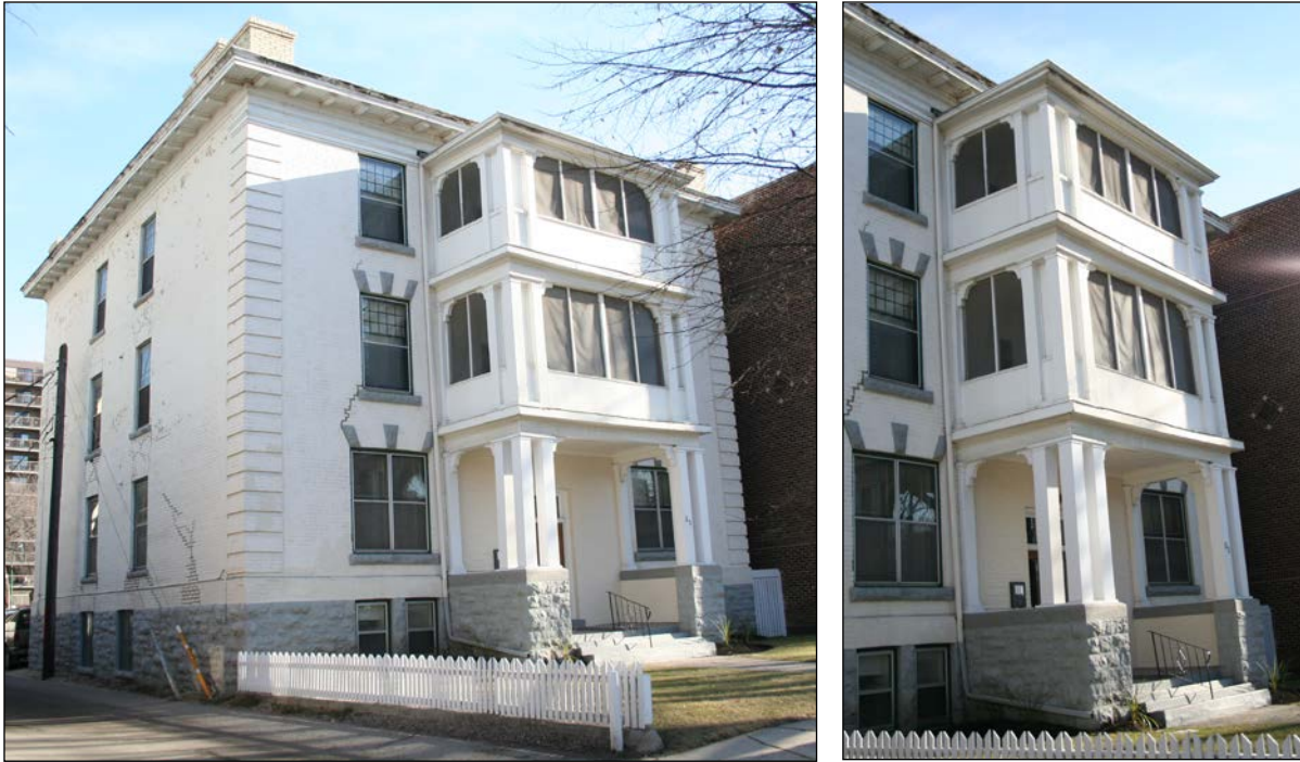
Front (west) and north façades (left) and front entrance detail (right), 2006
