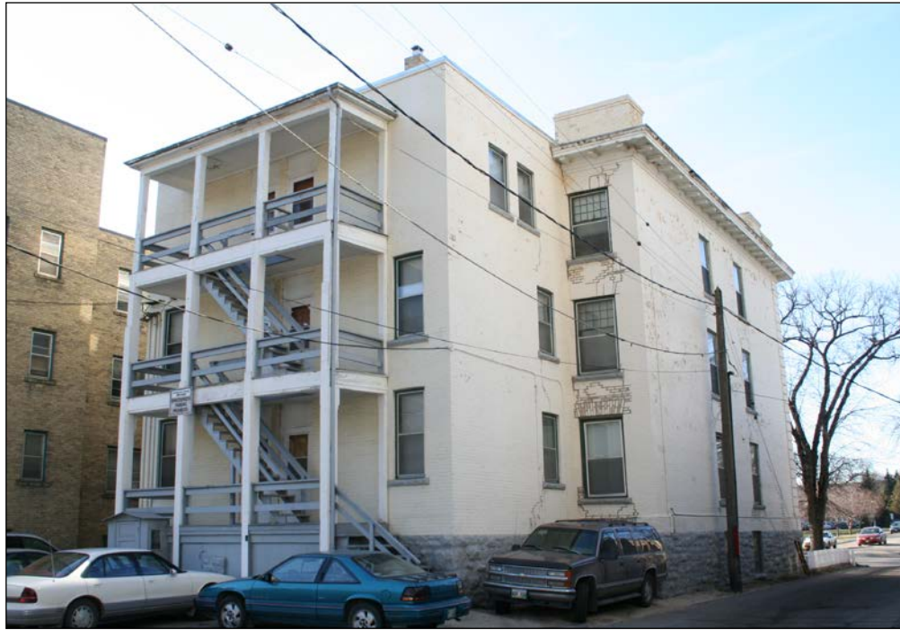
Rear (east) and north façades, 2006
