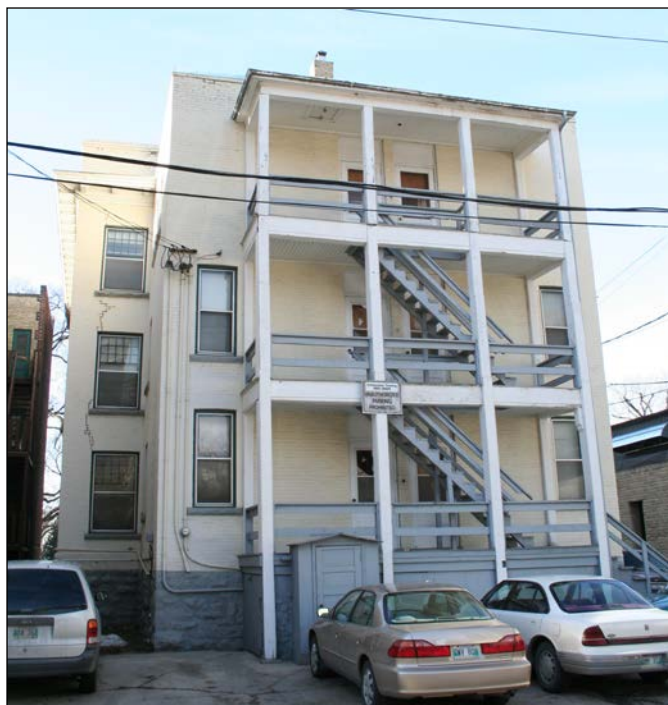
Rear (east) and south façades, 2006
