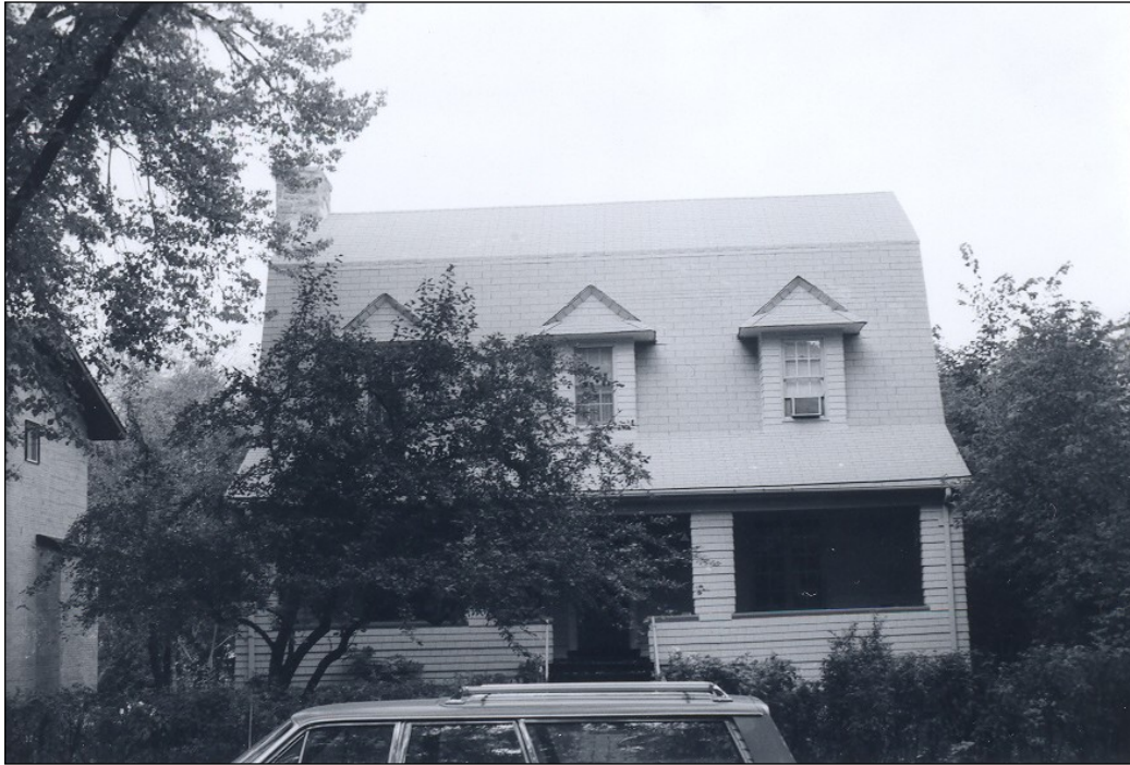
Front (south) façade, 1978
