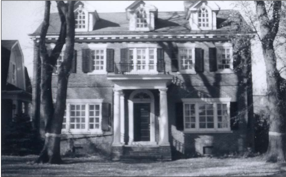
Front (south) façade, 1978
