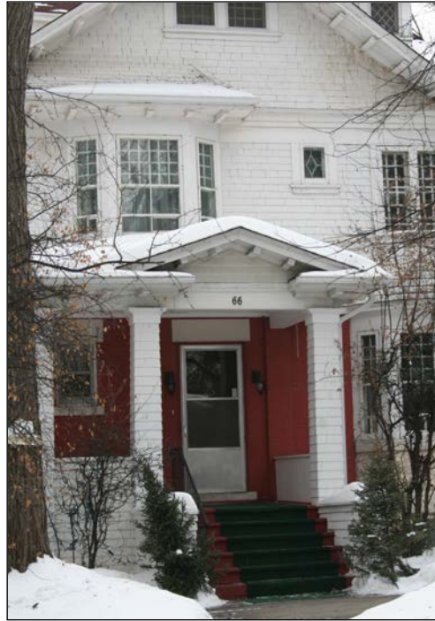
Front (north) façade detail, 2009
