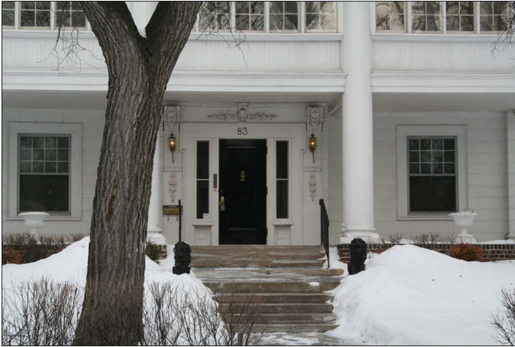
Front (south) façade detail, 2009
