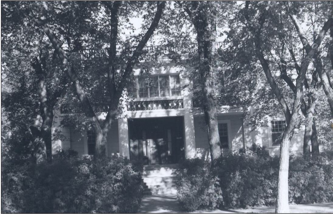
Front (south) façade detail, 1978
