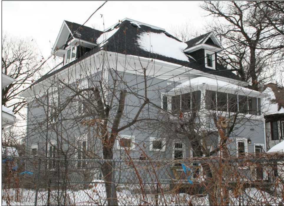
Rear (north) east façades, 2009
