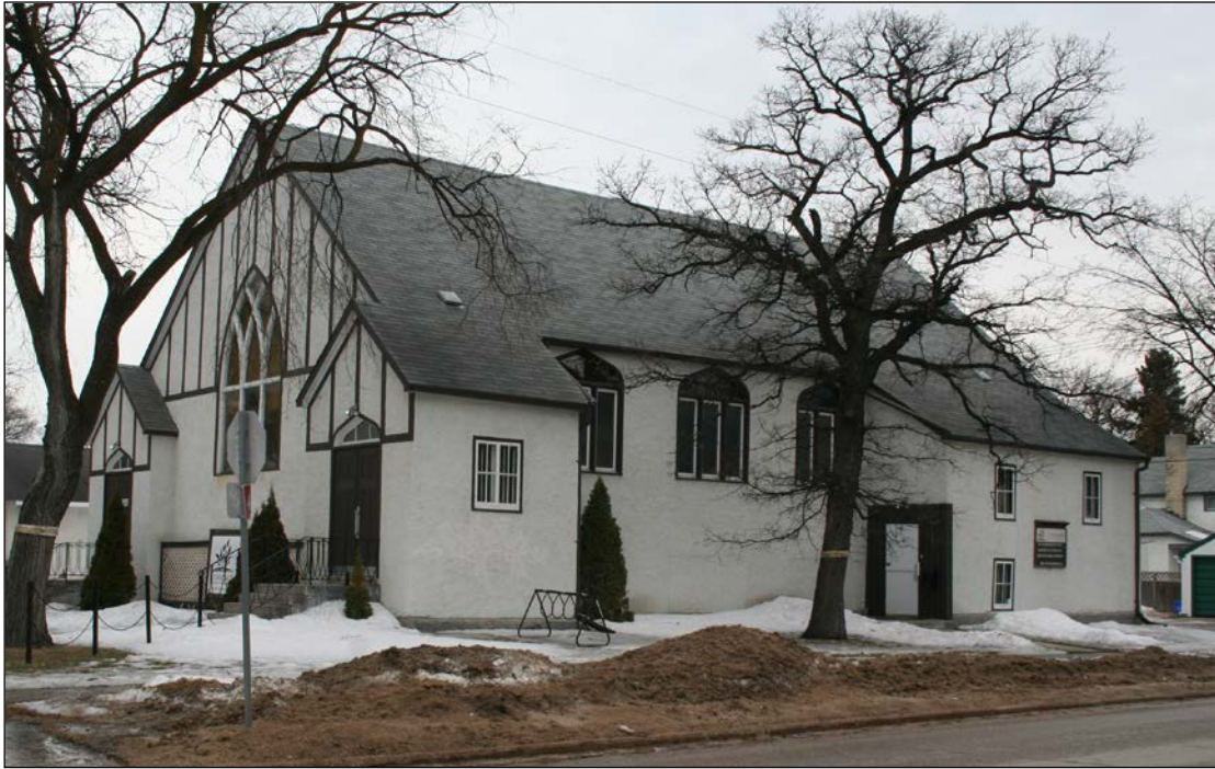
Front (south) and east façades, 2009
