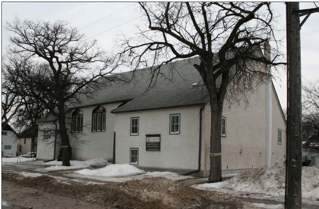
Rear (north) and east façades, 2009
