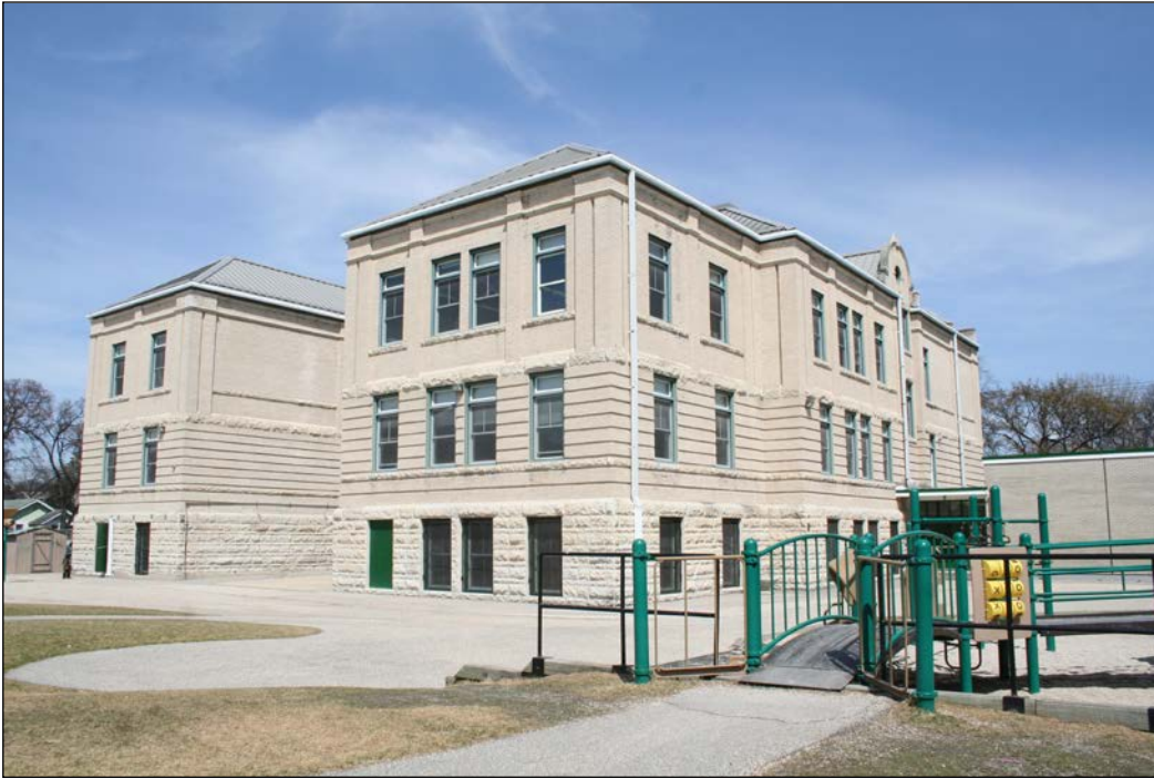
Rear (west) and south façades, 2009
