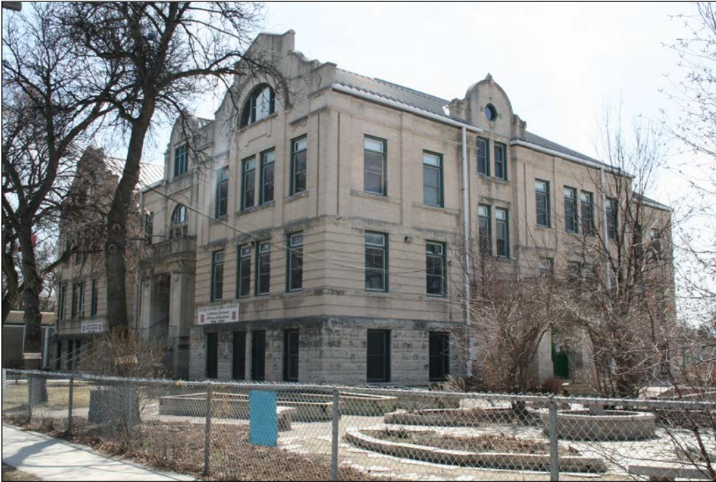
Front (east) and north façades, 2009
