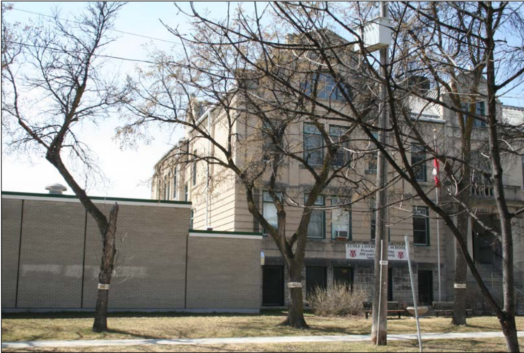
Front (east) and south façades, 2009
