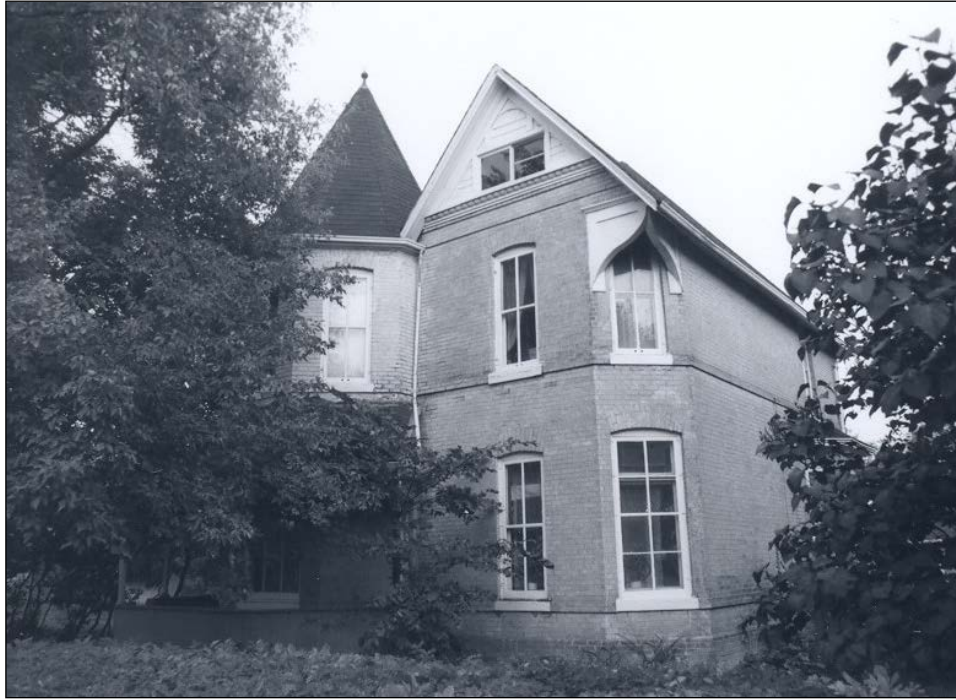
Front (west) façade, 1978
