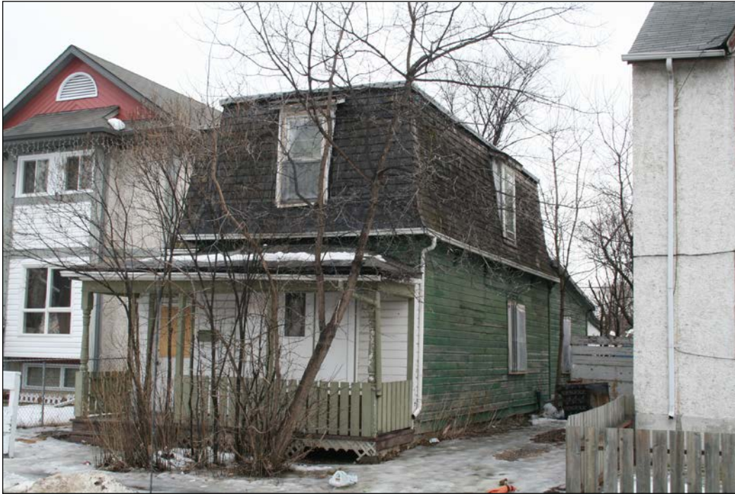
Front (south) and east façades, 2009
