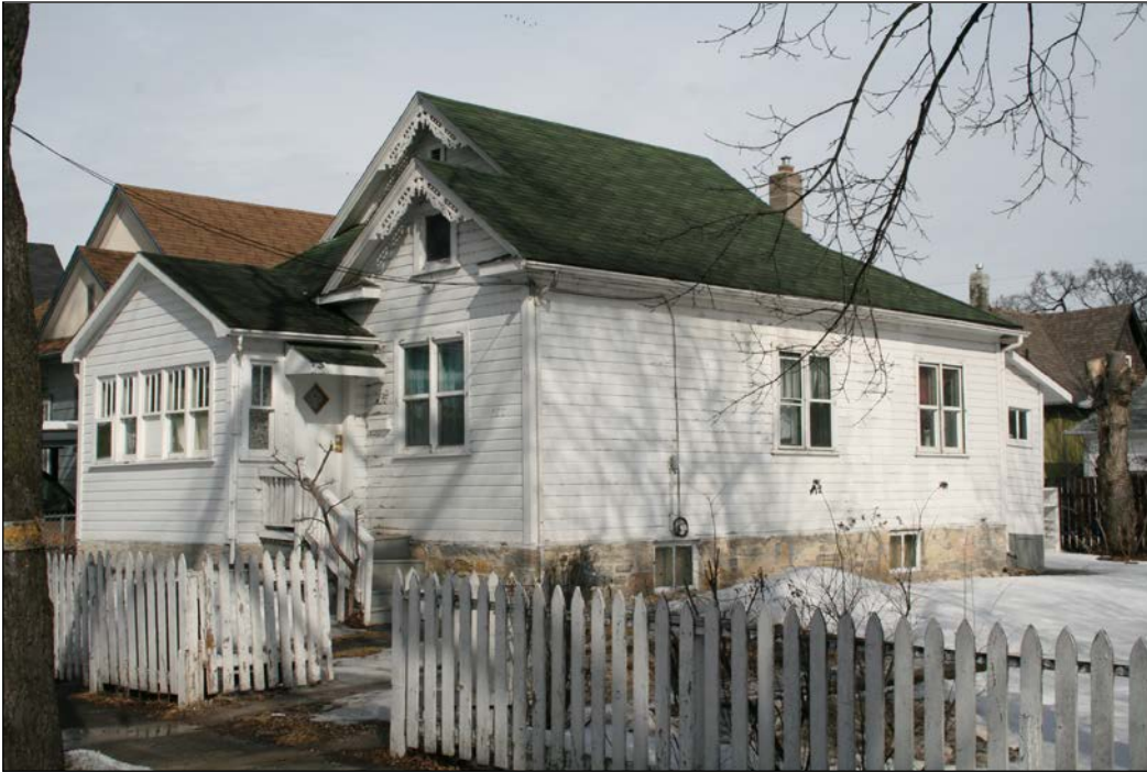
Front (south) and east façades, 2009
