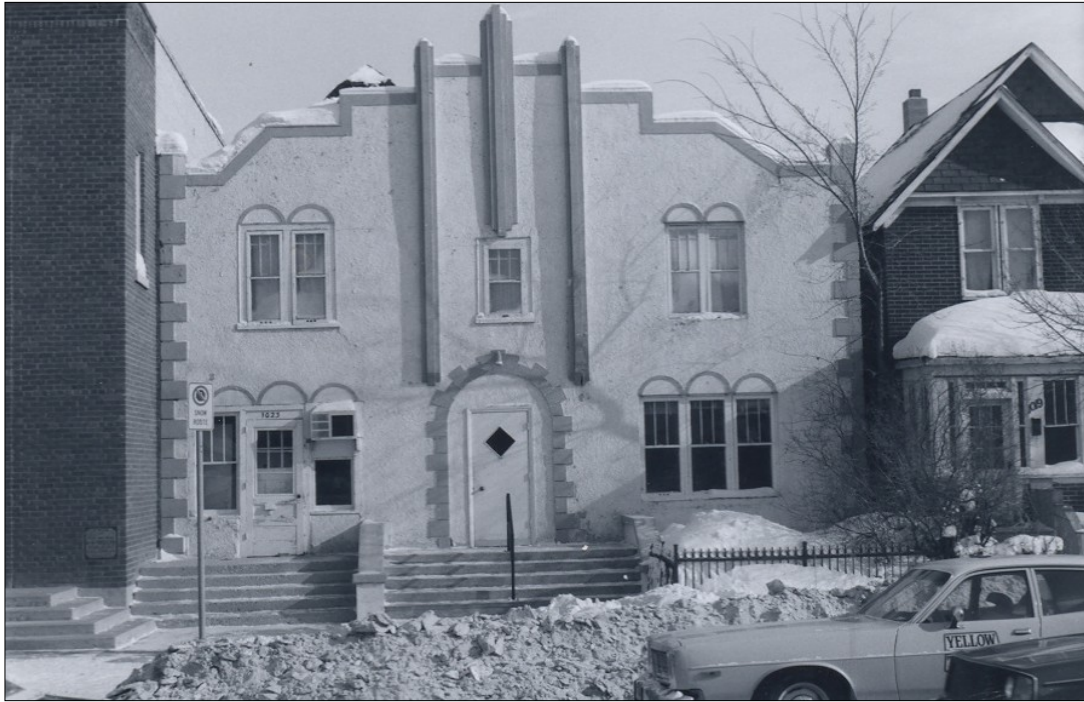
Front (west) façade, 1978
