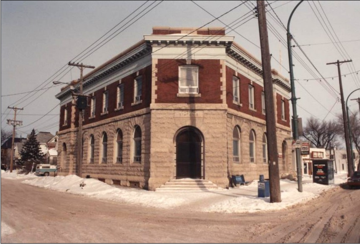
4 Postal Station "B", 1048 Main Street; built 1907, chief architect D. Ewart, contractor J. McDiarmid Company; south and east facades. ( Murray Peterson, 1992. )
