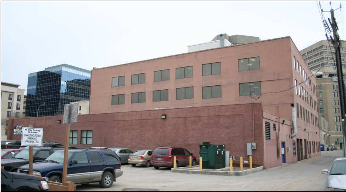
Rear (east) and south façades, 2006
