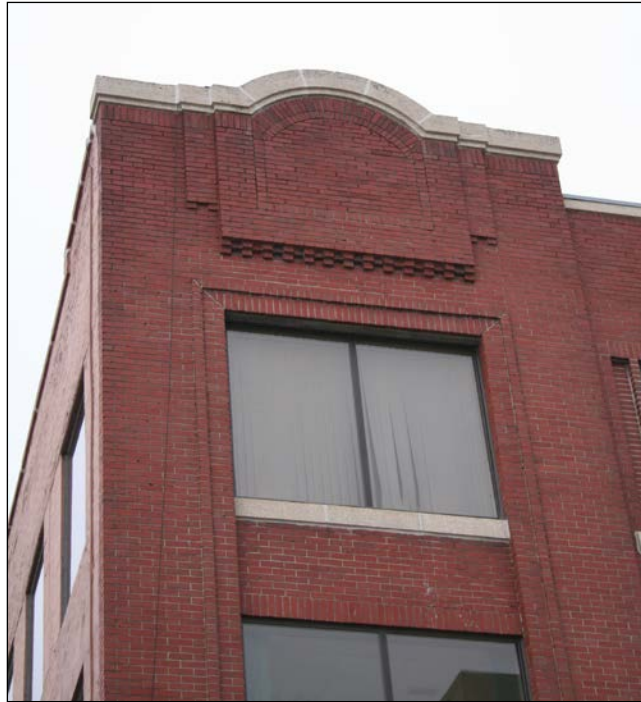
Northeast corner detail, 2006
