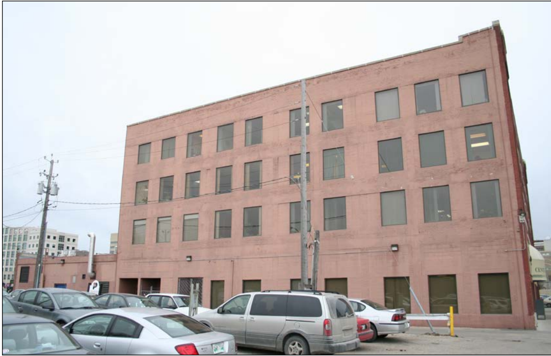
Rear (east) façade, 2006
