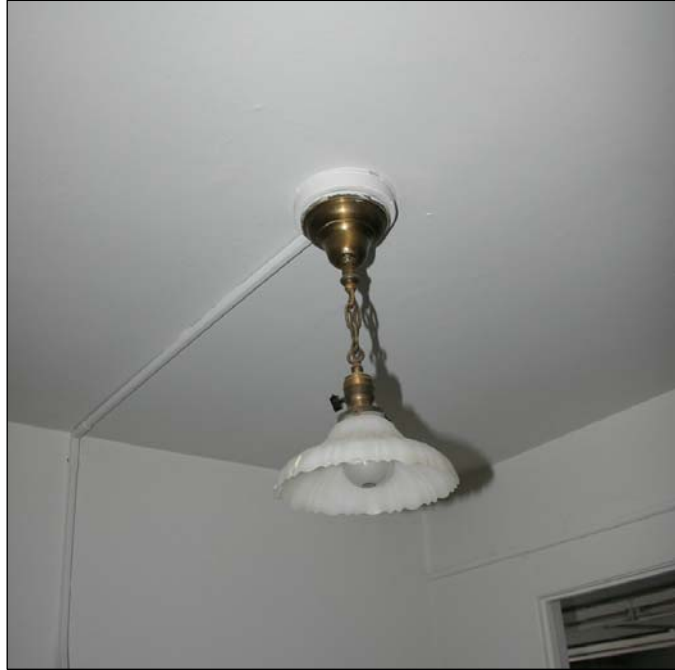
Plate 31 – Scott Block, 272 Main Street, mezzanine light fixture, 2010. ( M. Peterson, 2010. )
