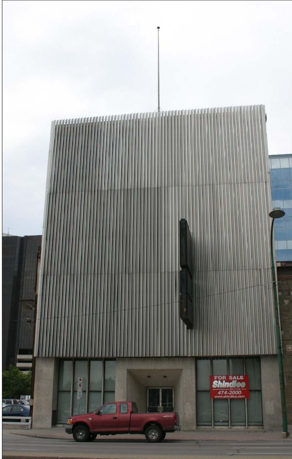
Plate 21 – Scott Block, 272 Main Street, front (east) façade, with the metal cladding and the smooth-cut limestone ground floor and newer entrance and windows, 2010. ( M. Peterson, 2010. )
