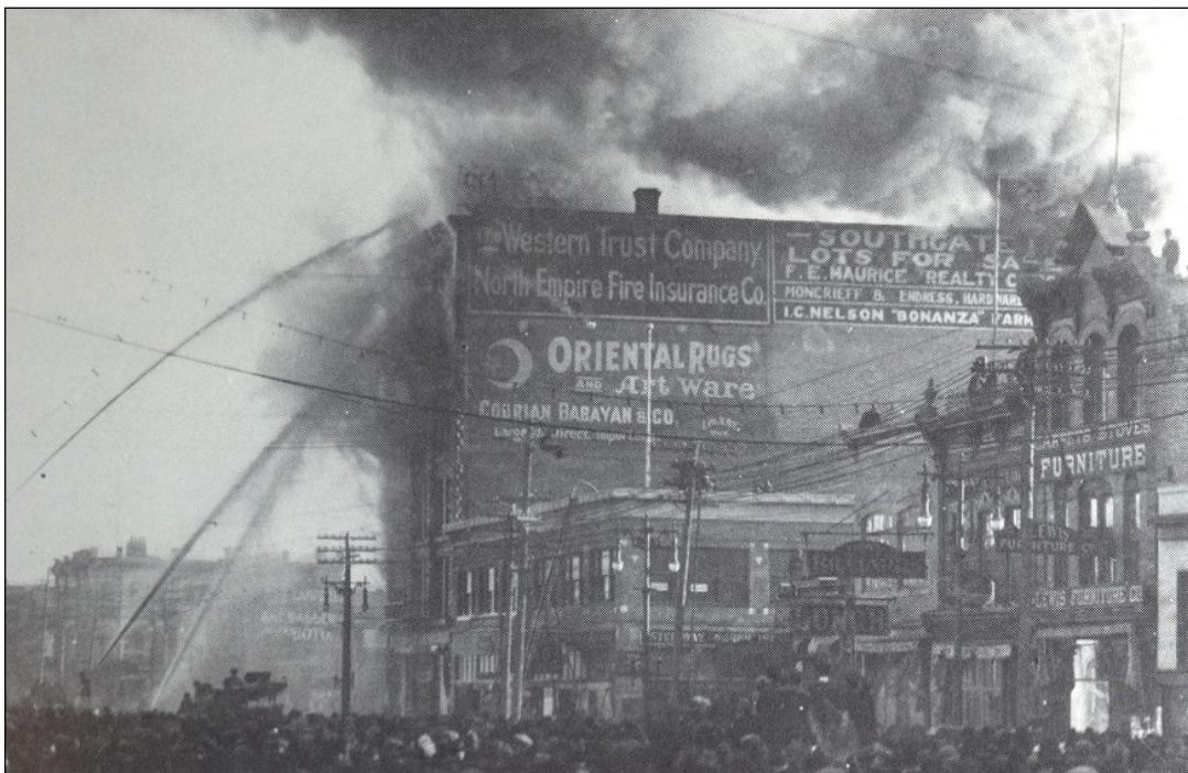
Plate 12 – 1915 fire at the Scott Block, 272 Main Street, March 23, 1914. ( Reproduced from V. Leah, Alarm of Fire (Winnipeg, MB: Firefighters Burn Fund, 1982), p. 75. )
