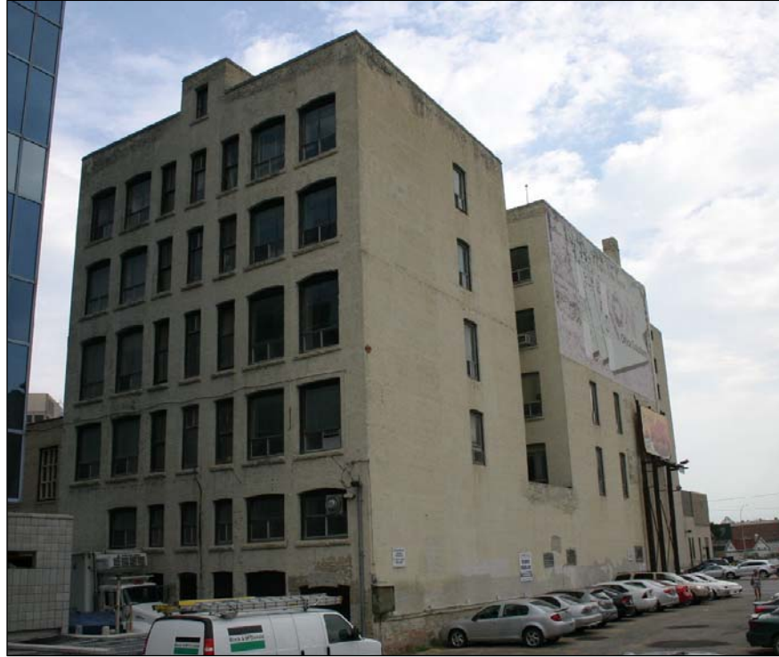
Plate 18 – Scott Block, 272 Main Street, rear (west) and south façades, 2010. ( M. Peterson, 2010. )
