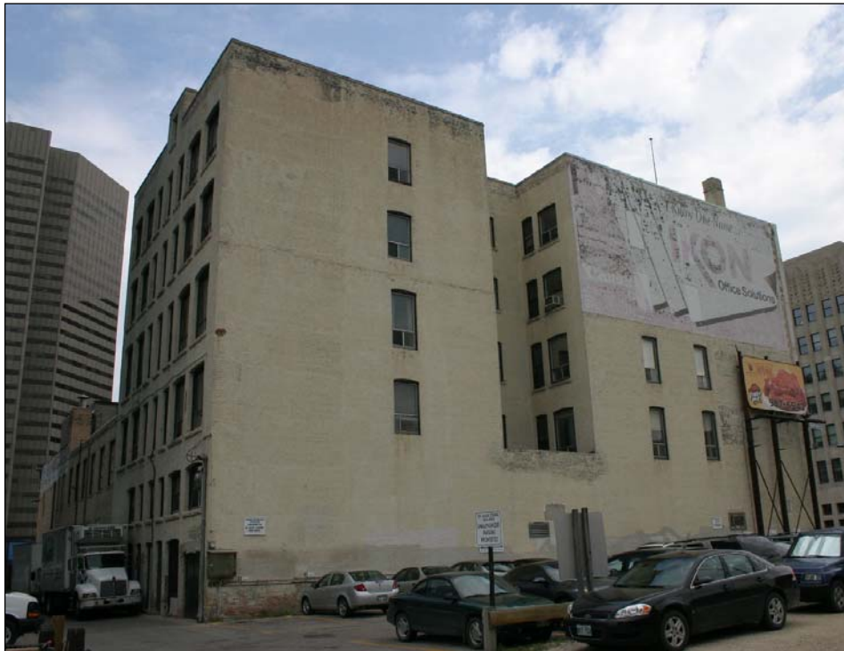
Plate 19 – Scott Block, 272 Main Street, south façade, 2010. ( M. Peterson, 2010. )
