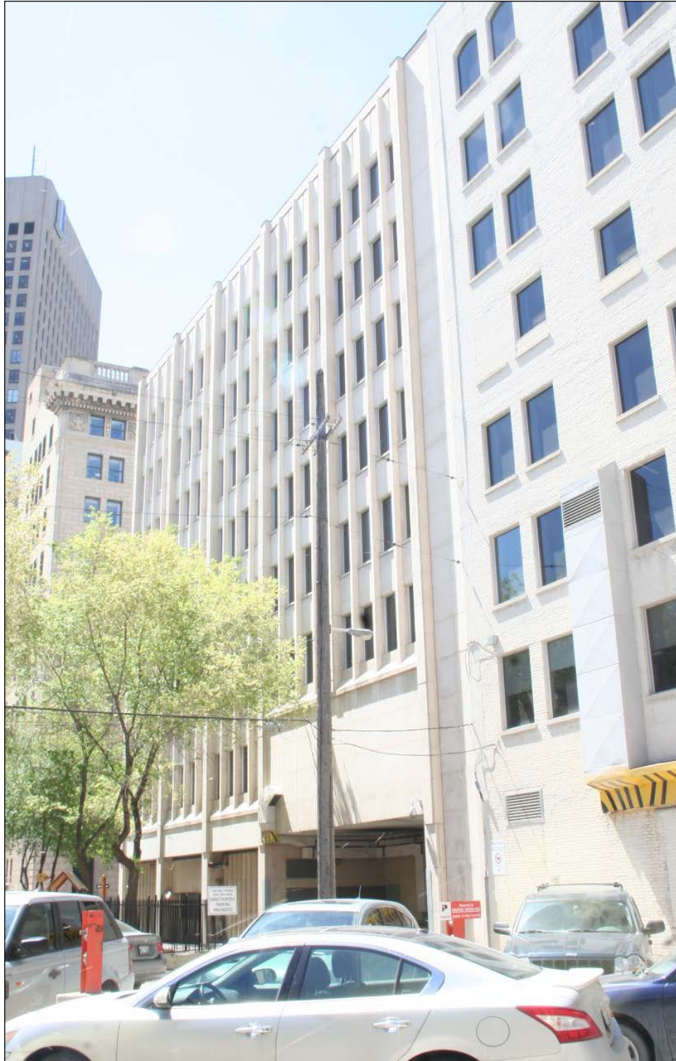
Plate 24 – Canadian Wheat Board Building, 423 Main Street, rear (east) façade of 1962-1964 addition, 2014. (M. Peterson, 2014.)
