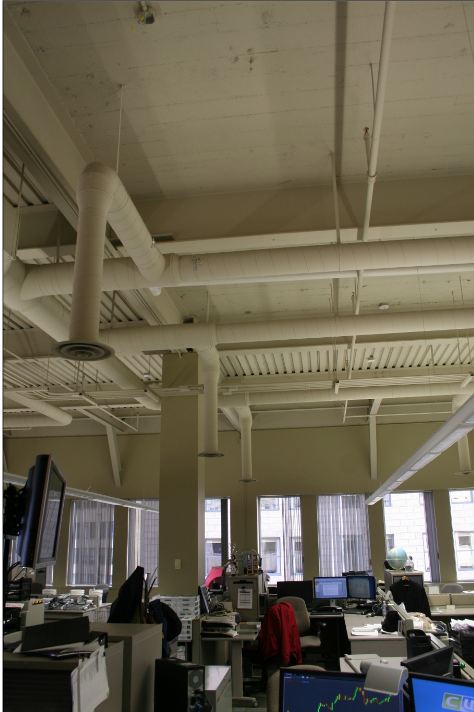
Plate 26 – Canadian Wheat Board Building, 423 Main Street, 8 th floor office space with high ceilings, 2014. (M. Peterson, 2014.)
