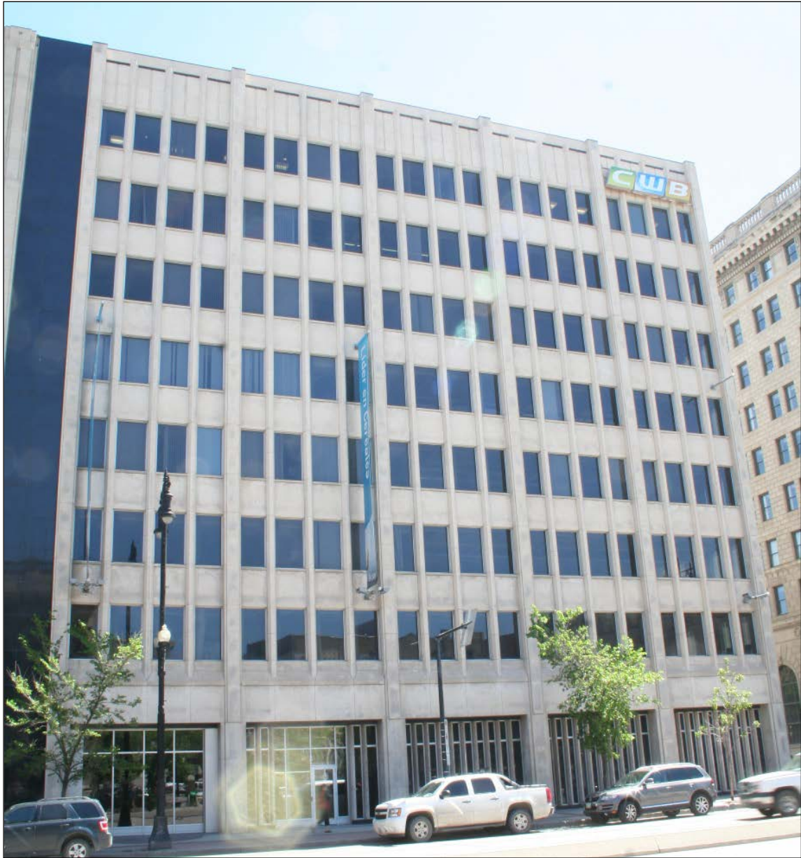
Plate 20 – Canadian Wheat Board Building, 423 Main Street, front (west) façade of 1962-1964 addition, 2014. (M. Peterson, 2014.)
