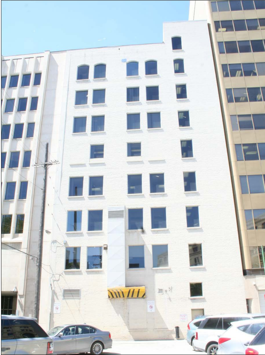
Plate 19 – Canadian Wheat Board Building, 423 Main Street, rear (east) façade, 2014. ( M. Peterson, 2014. )
