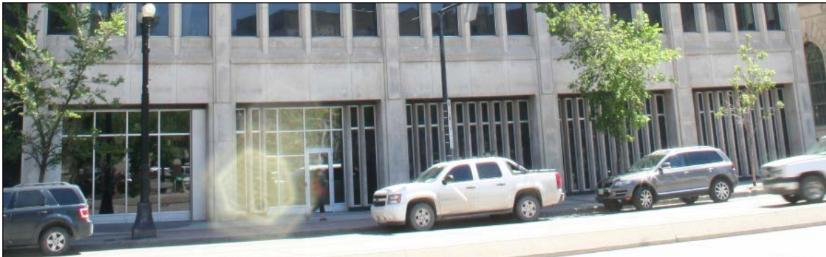
Plate 22 – Canadian Wheat Board Building, 423 Main Street, detail of ground floor of front (west) façade of 1962-1964 addition, 2014. ( M. Peterson, 2014. )
