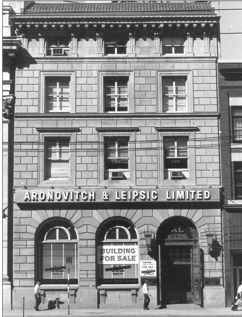
Plate 3 – Royal Bank, 460 Main Street, front façade, 1970. ( Courtesy of the Provincial Archives of Manitoba, Architectural Survey. )
