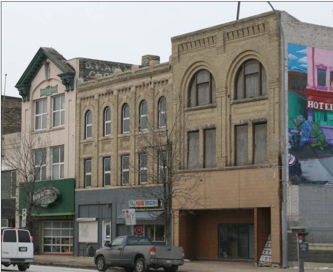
Plate 7– Guest Block, 598 Main Street, and neighbouring buildings, 2014. (M. Peterson, 2014.)
