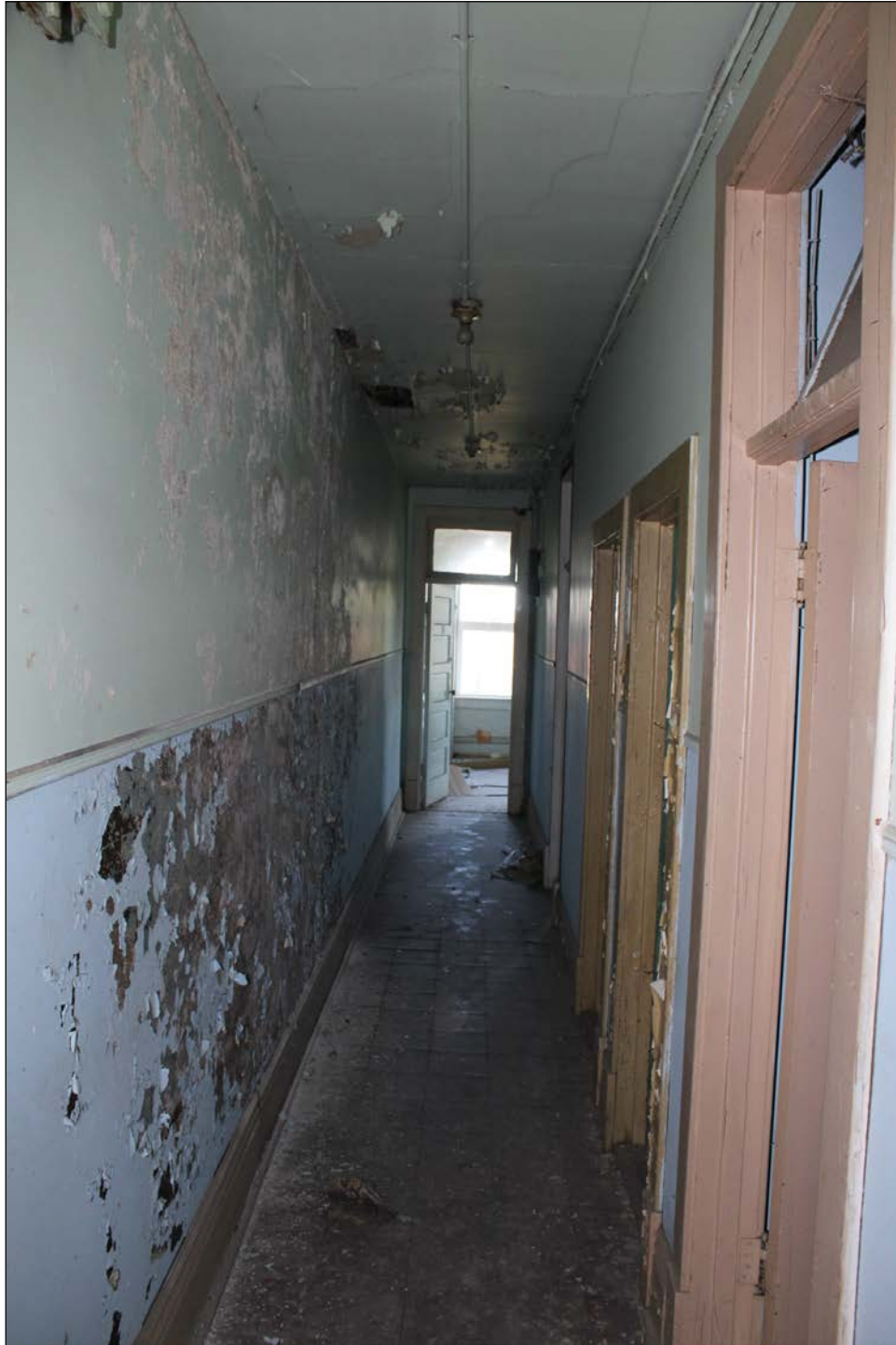
Plate 11 – Guest Block, 598 Main Street, third floor hallway, 2015. ( M. Peterson, 2015. )
