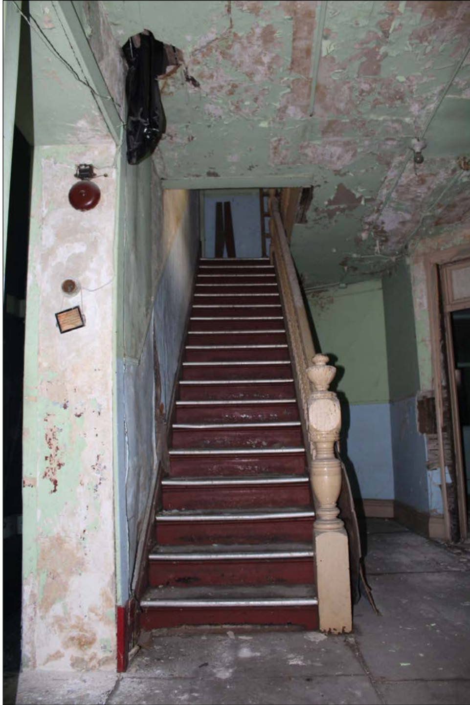
Plate 10 – Guest Block, 598 Main Street, stairs to third floor, 2015. ( M. Peterson, 2015. )
