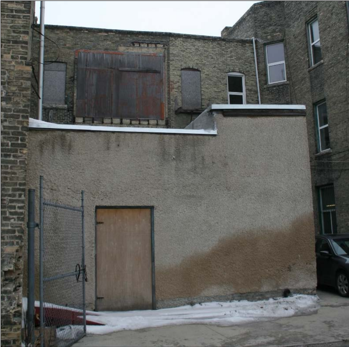
Plate 8 – Guest Block, 598 Main Street, rear (west) façade, 2014. ( M. Peterson, 2014. )
