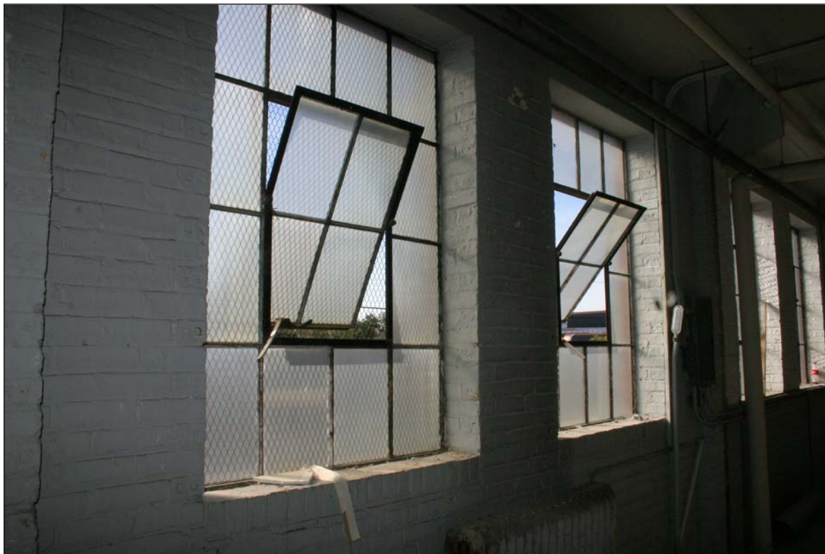
Plate 9 – 765 Main Street, Canadian Pacific Railway Post Office Building, second storey industrial windows with opened panes, 2011. ( M. Peterson, 2011. )
