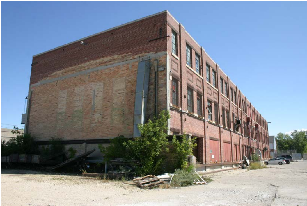
Plate 1 – 765 Main Street, Canadian Pacific Railway Post Office Building, south and west facades, 2011. (M. Peterson, 2011.)
