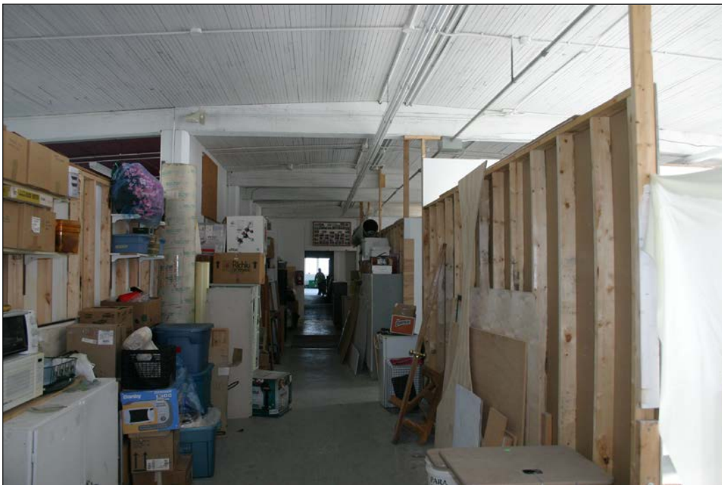
Plate 13 – 765 Main Street, Canadian Pacific Railway Post Office Building, third floor, 2011. ( M. Peterson, 2011. )
