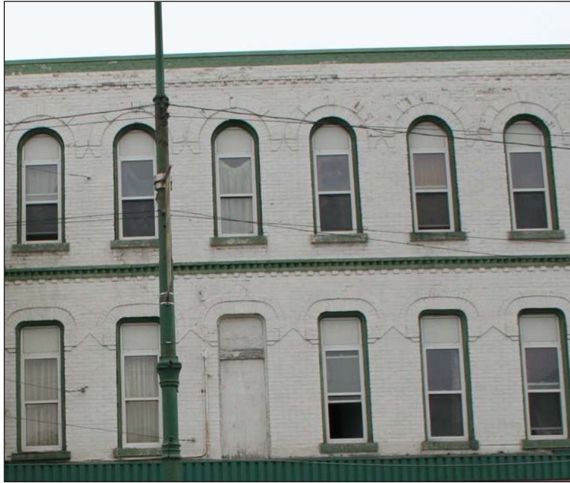
Front (east) façade detail, 2009
