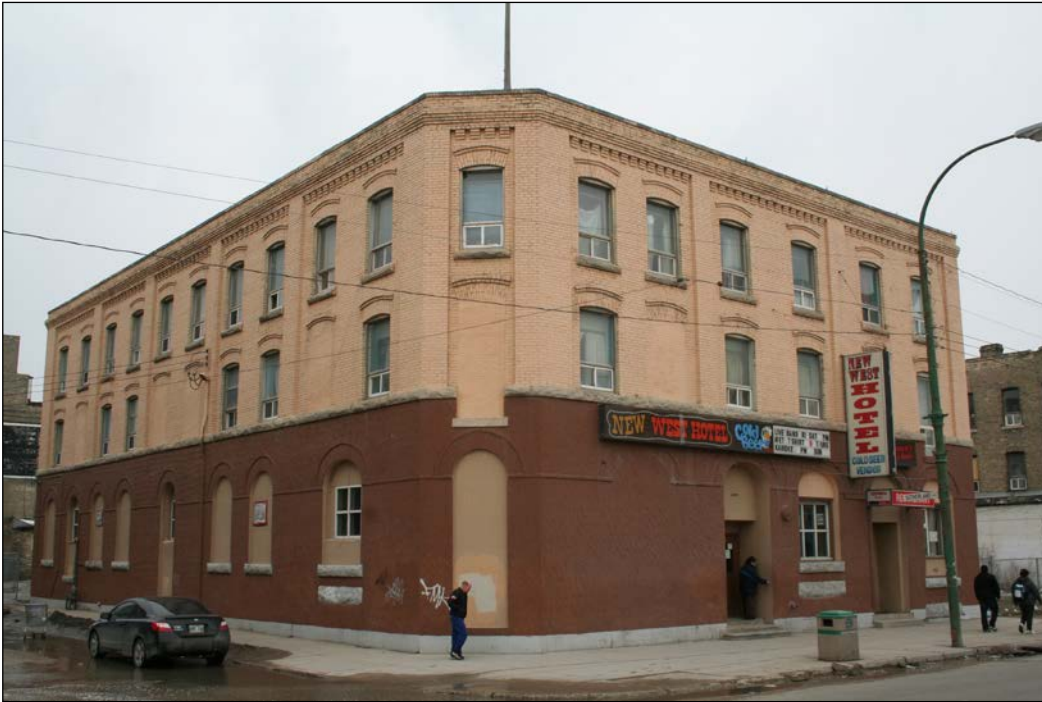
Front (east) and south façades, 2009
