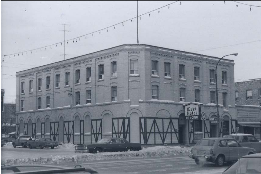
Front (east) and south façades, 1978
