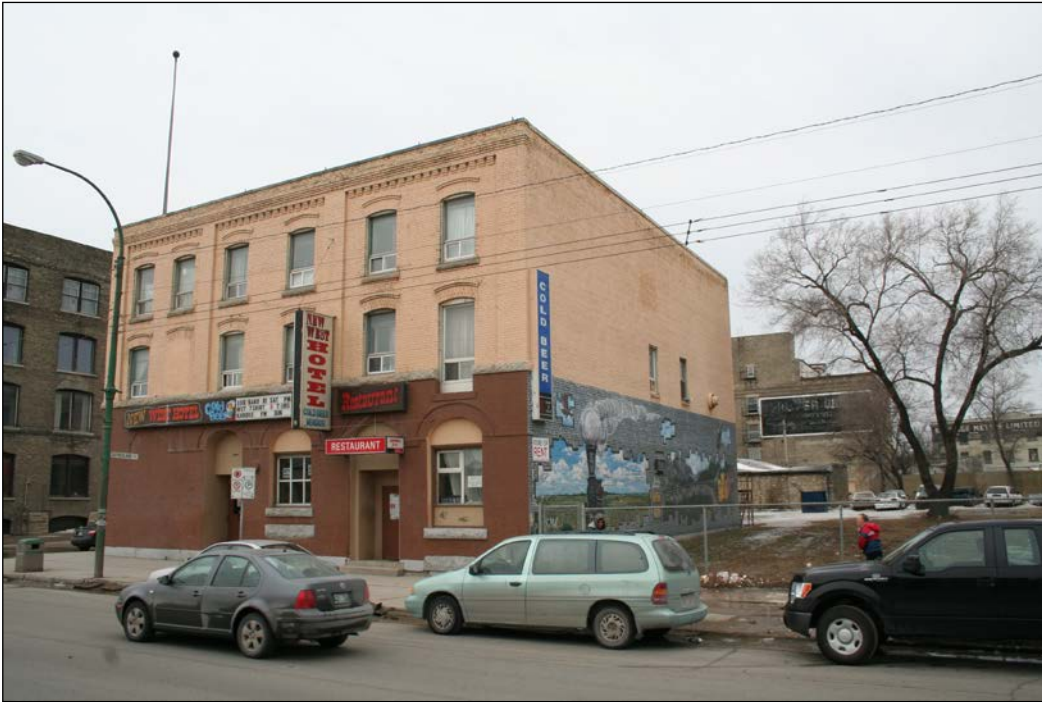
Front (east) and north façades, 2009
