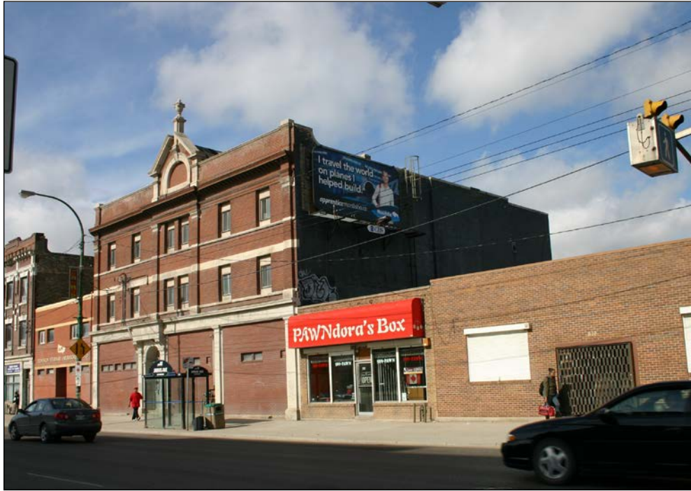
Front (east) and north façades, 2009
