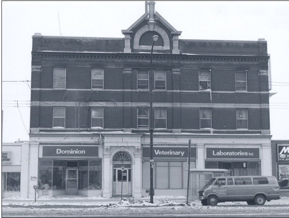
Front (east) façade detail, 1978
