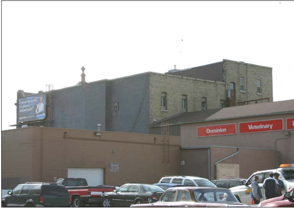
Rear (west) and north façades, 2009
