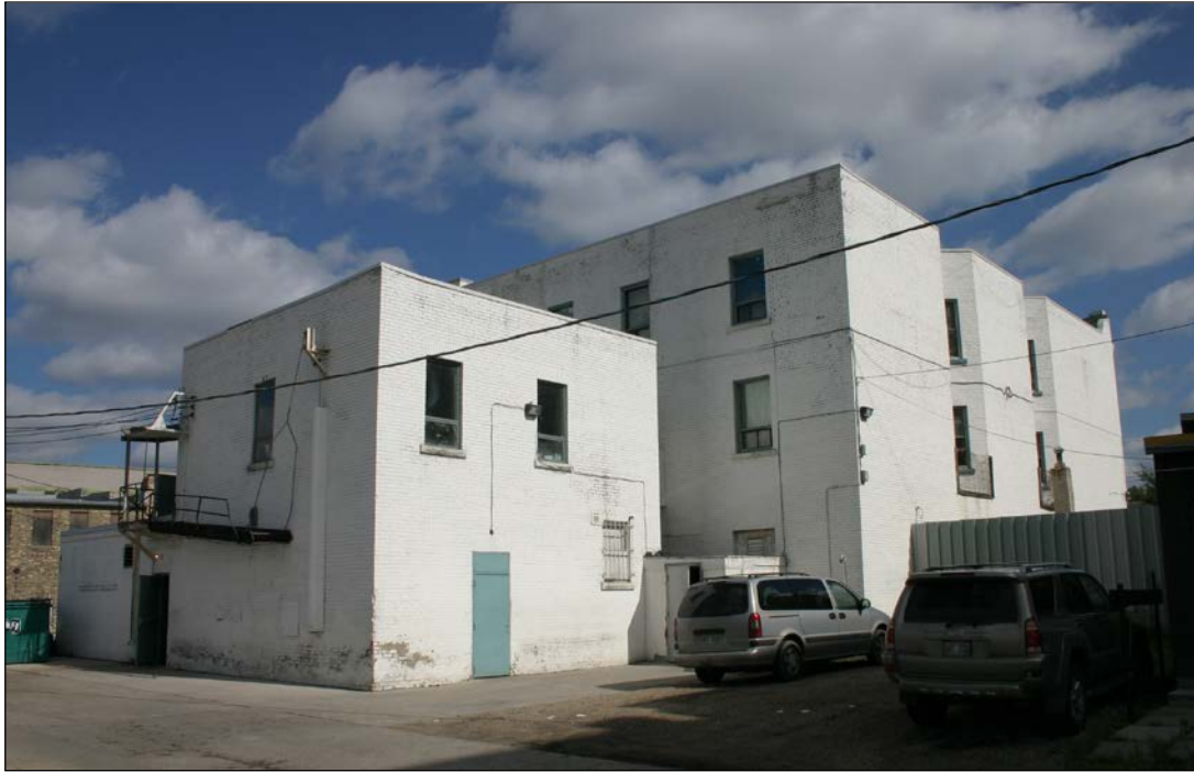
Rear (west) and south façades, 2005
