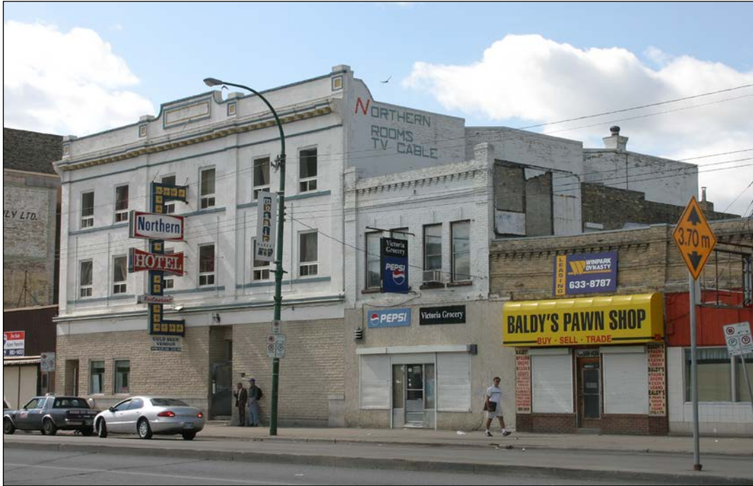
Front (east) and north façades, 2005
