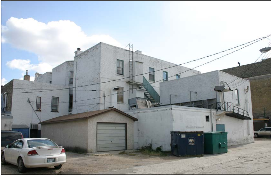
Rear (west) and north façades, 2005
