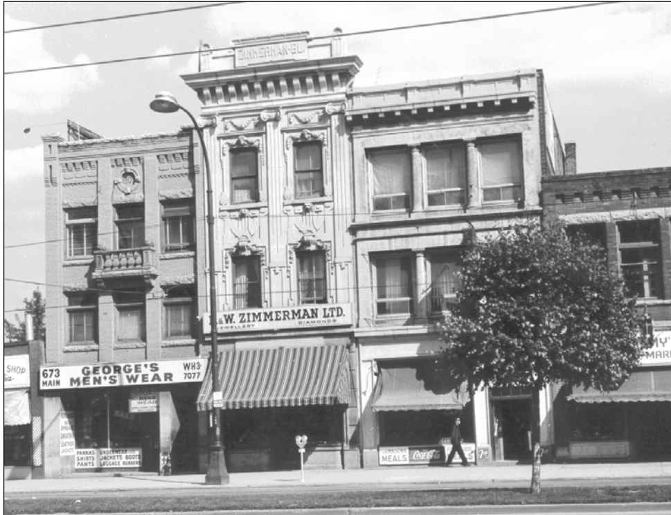
Plate 1 – 667-73 Main Street, the Alloway and Champion Building is three-storey building partially hidden by the tree, 1969. (Courtesy of the Provincial Archives of Manitoba, Architectural Survey.)
