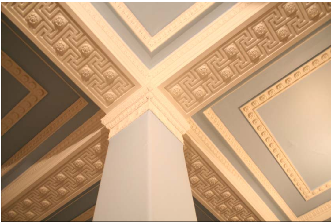
Plate 21 – Dominion Bank, 678 Main Street, portion of banking hall ceiling. ( M. Peterson, 2006. )
