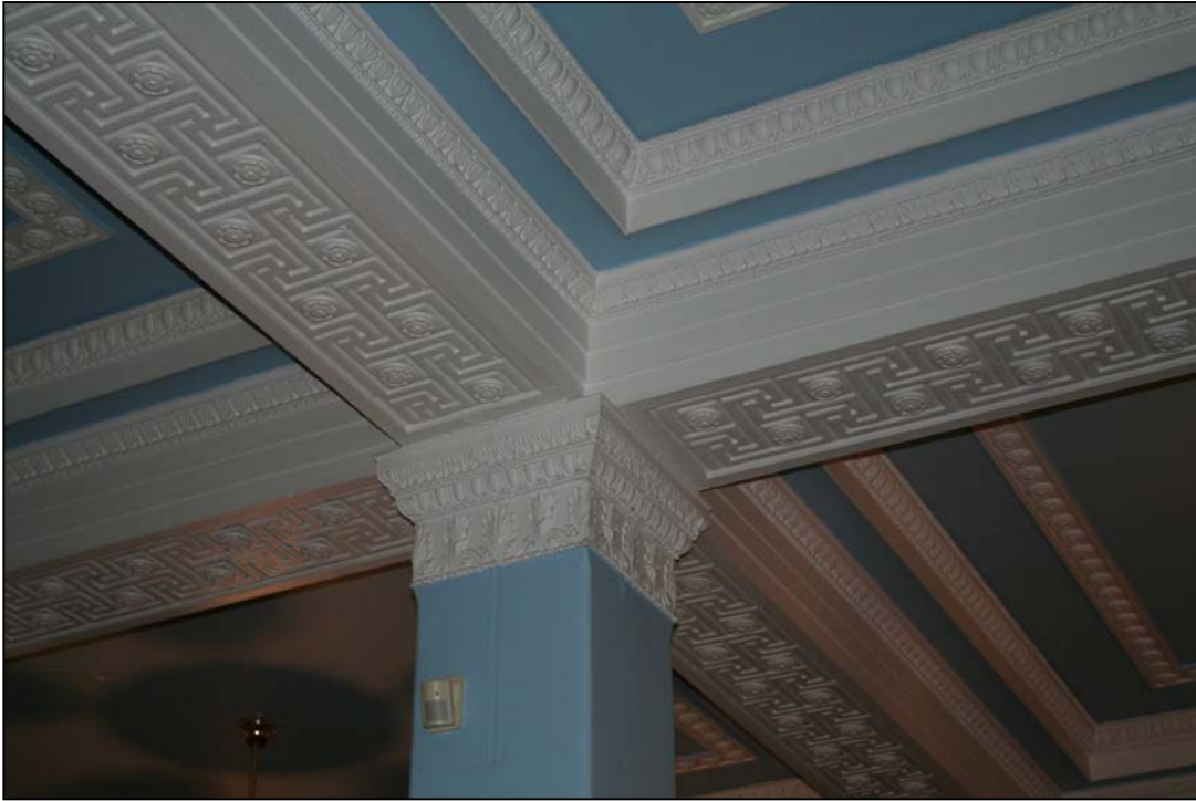
Plate 20 – Dominion Bank, 678 Main Street, portion of banking hall ceiling. ( M. Peterson, 2006. )
