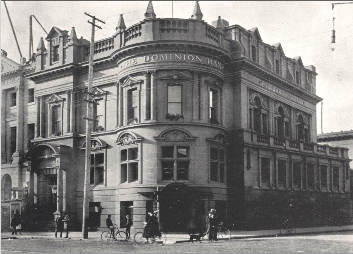
Plate 29 – Dominion Bank, 440 Main Street (southwest corner McDermot Avenue), ca.1903; constructed 1898-99, designed by Darling and Pearson. ( Reproduced from Illustrated Souvenir of Winnipeg [Winnipeg: Wm. A. Martel & Sons, ca.1903], p. 183. )
