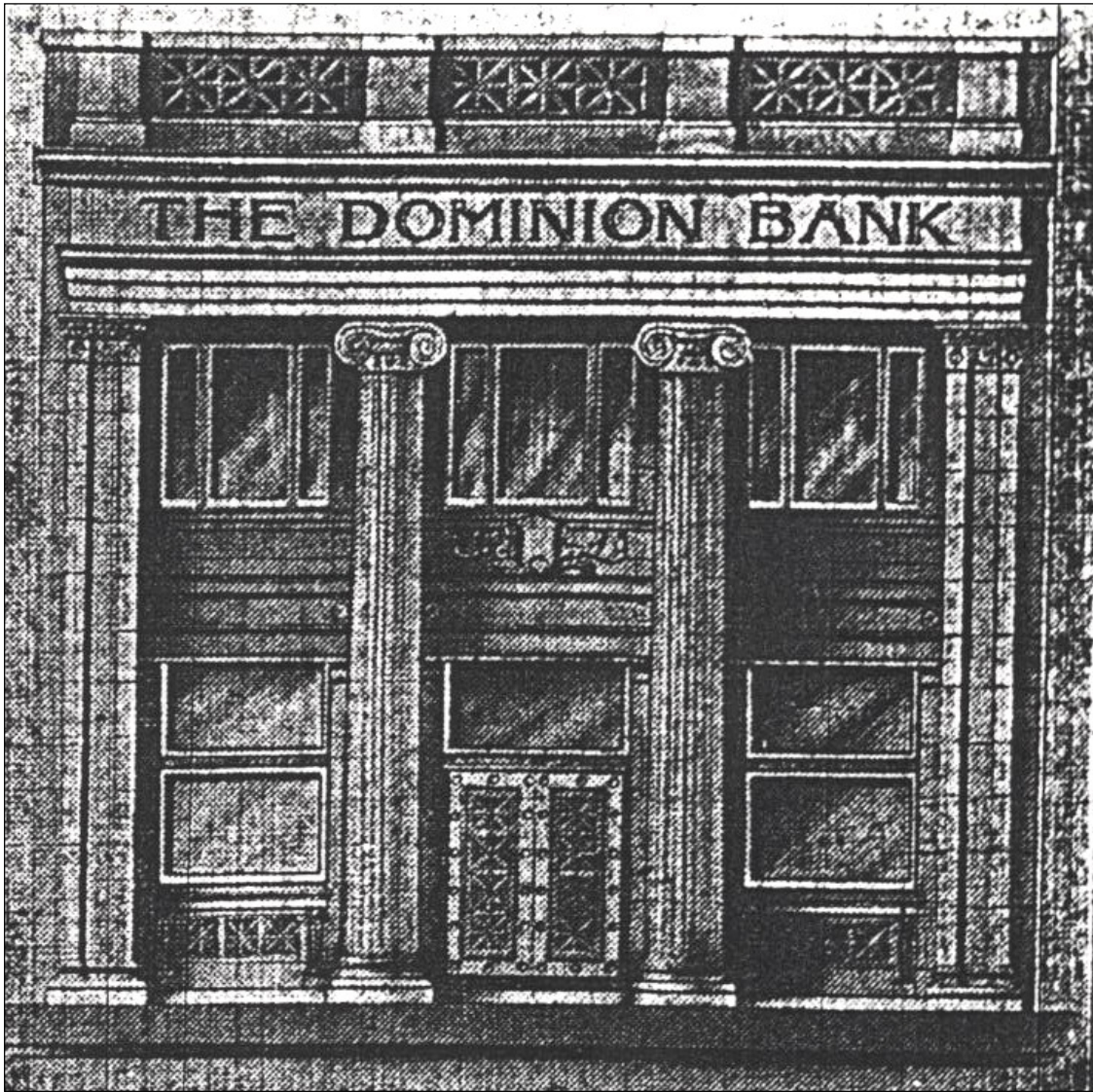
Plate 6 – The Dominion Bank, 678 Main Street, as it was built in 1907. The original windows were paired on the ground floor and triplets on the second floor and the original entrance door included transom window and ornamental metal grating. (Reproduced from Manitoba Free Press , January 25, 1908, p. 5.)
