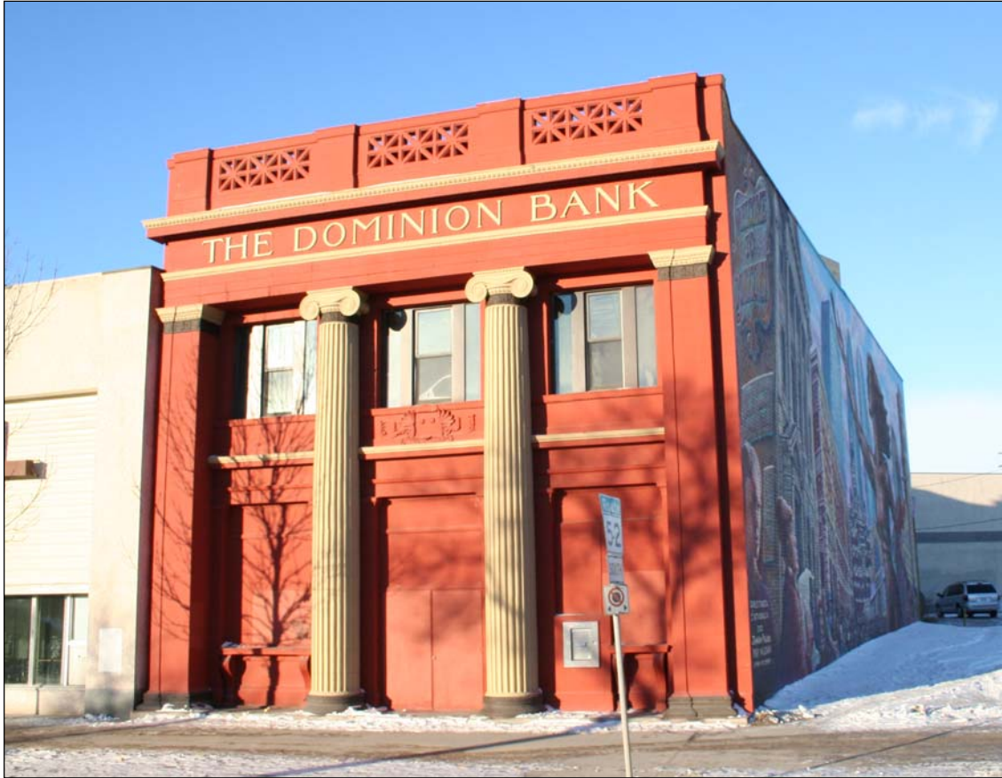
Plate 3 – Dominion Bank, 678 Main Street, front (east) and north façades. (M. Peterson, 2006.)
