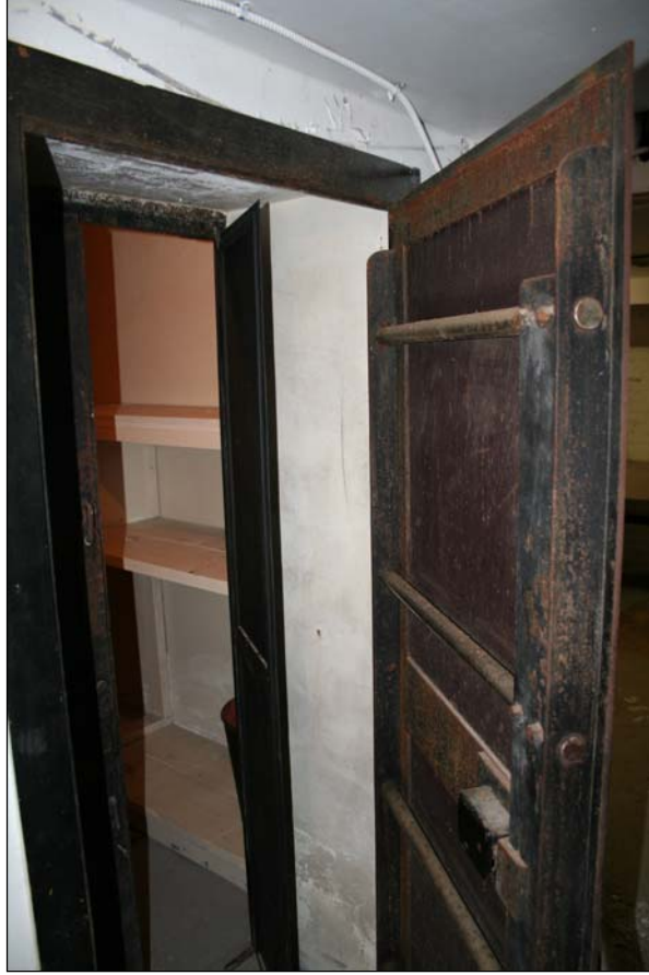
Plate 16 – Dominion Bank, 678 Main Street, basement walk-in vault. ( M. Peterson, 2006. )
