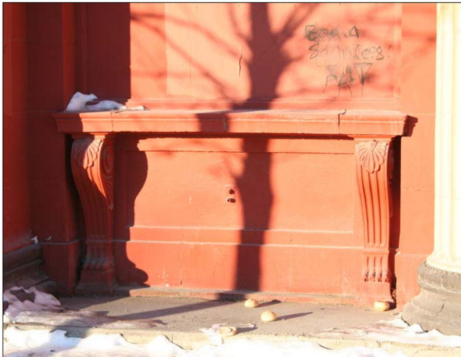
Plate 8 – Dominion Bank, 678 Main Street, detail of table-like sills on front façade. ( M. Peterson, 2006. )
