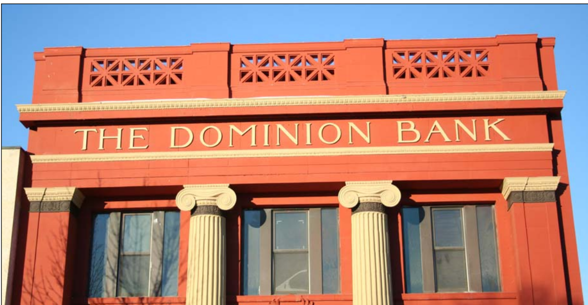
Plate 5 – Dominion Bank, 678 Main Street, detail of front façade. ( M. Peterson, 2006. )
