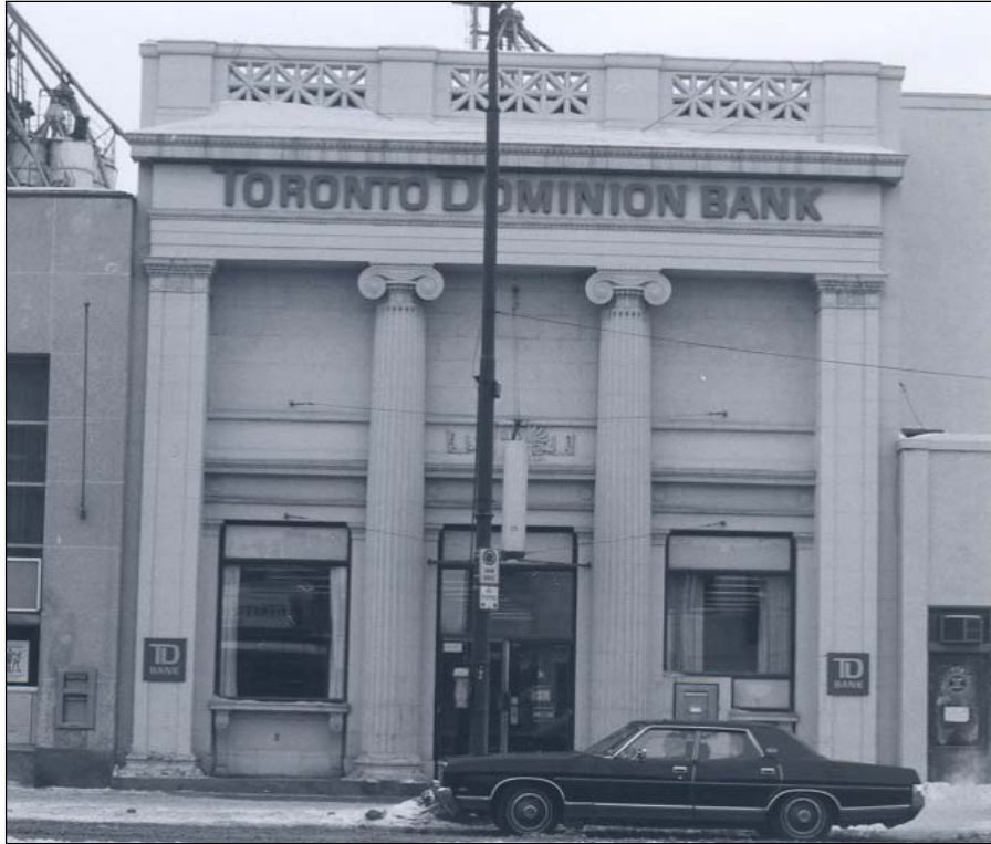
Plate 12 – Dominion Bank, 678 Main Street, front (east) façade, 1978, showing the altered ground floor window/door openings and the closed second storey window openings. ( City of Winnipeg, Historical Buildings Committee. )
