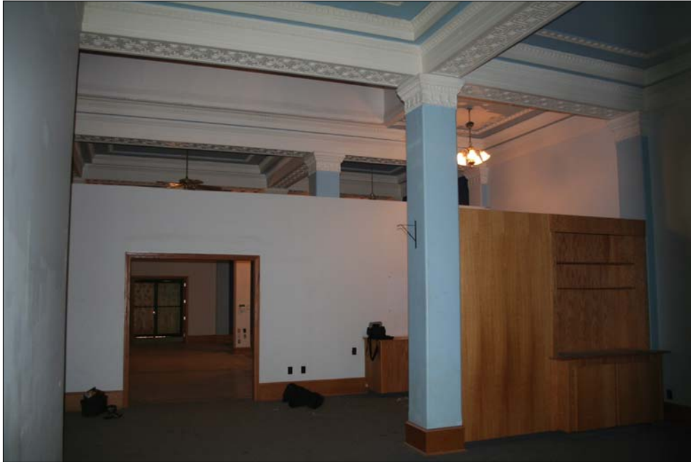
Plate 18 – Dominion Bank, 678 Main Street, main floor looking towards the front entrance foyer. (M. Peterson, 2006.)
