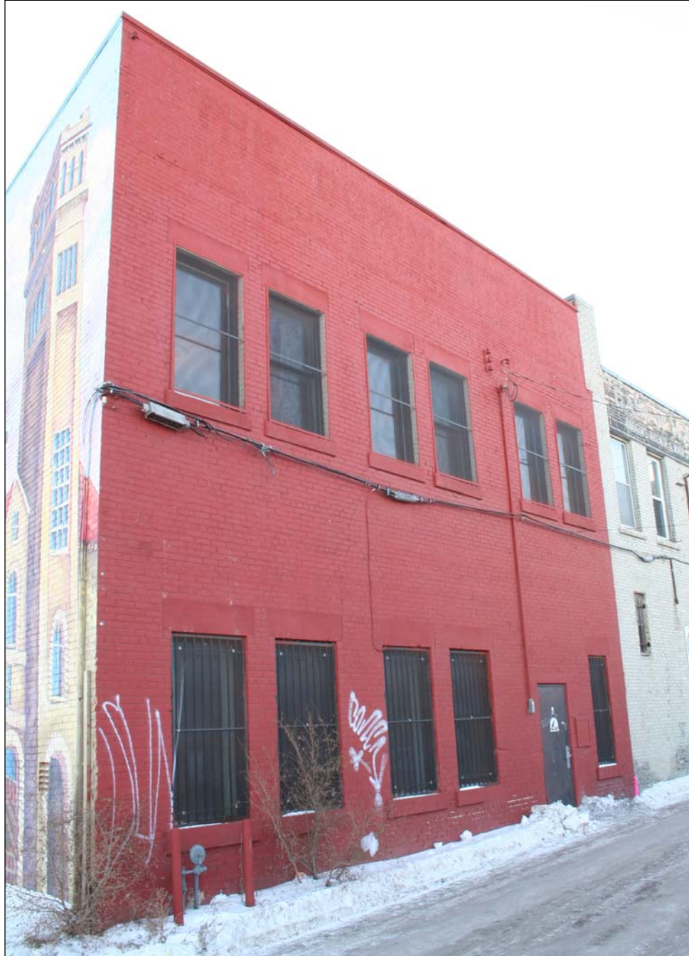
Plate 11 – Rear (west) façade. ( M. Peterson, 2006. )
