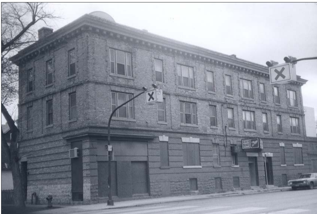
North and west façades, 1978
