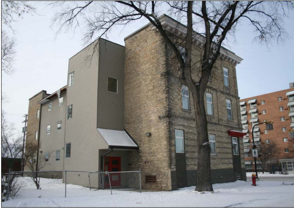
North and east façades, 2009
