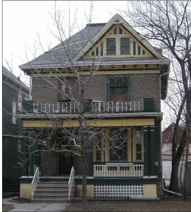
Front (east) façade, 2004
