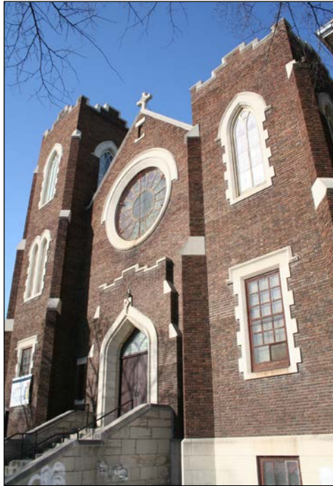
Front (east) façade detail, 2009
