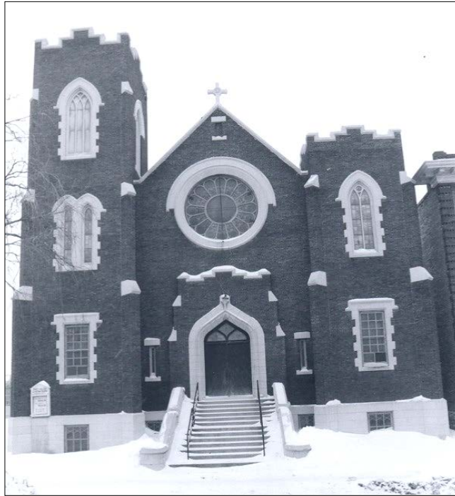
Front (east) façade detail, 1978
