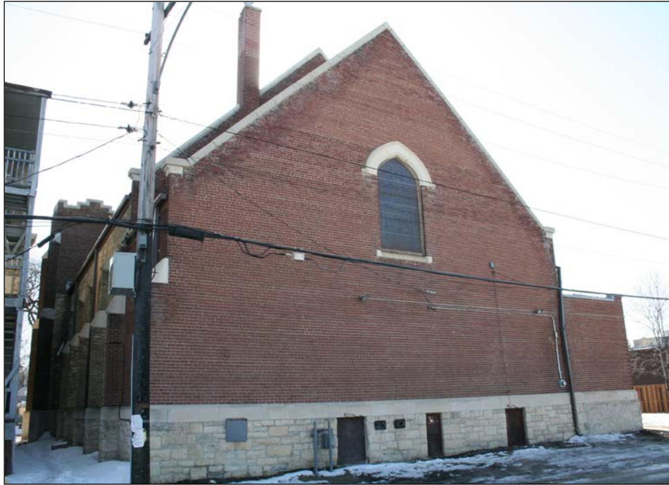
Rear (west) and north façades, 2009
