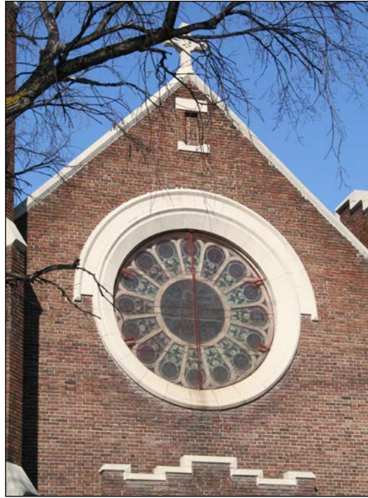
Front (east) façade rose window, 2009
