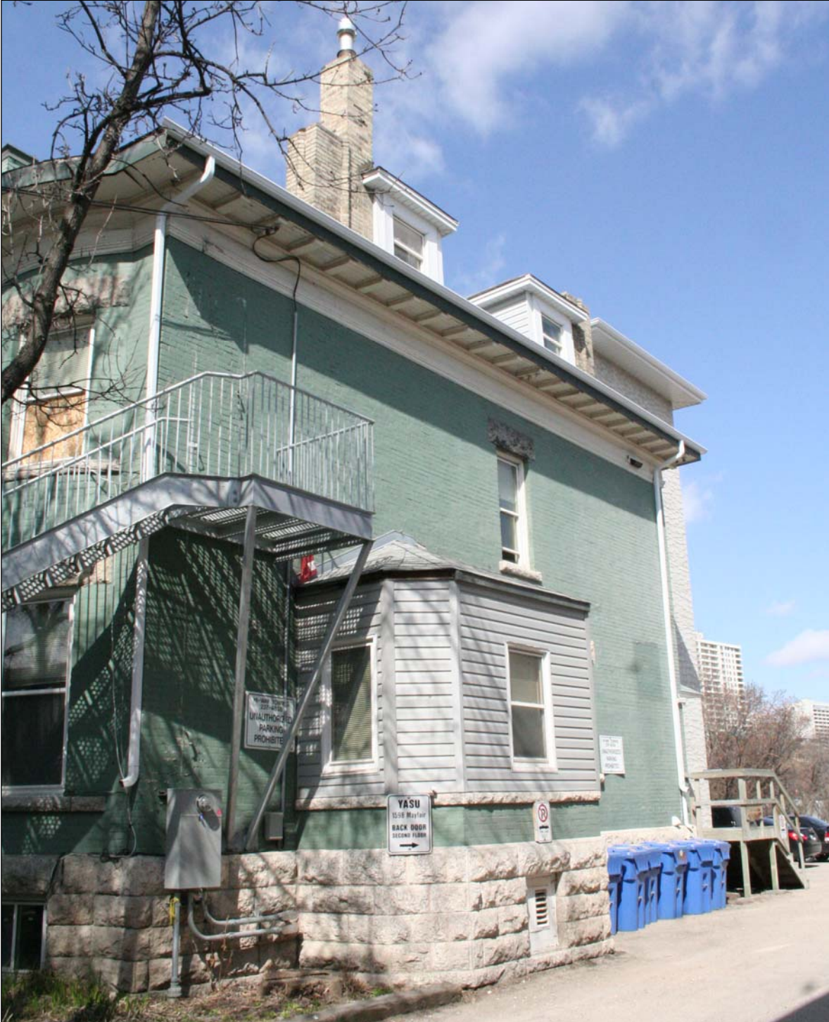
Plate 12 – 159 Mayfair Avenue, east façade, 2008. ( M. Peterson, 2008. )
