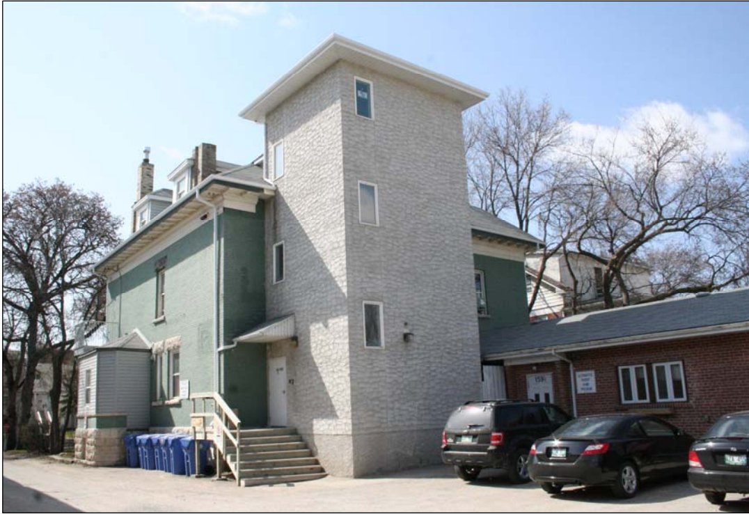
Plate 15 – 159 Mayfair Avenue, rear (north) and east façades, 2008. (M. Peterson, 2008.)
