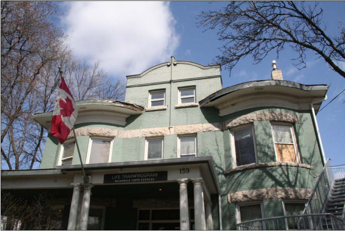
Plate 11 – 159 Mayfair Avenue, detail of front (south) elevation, 2008. ( M. Peterson, 2008. )
