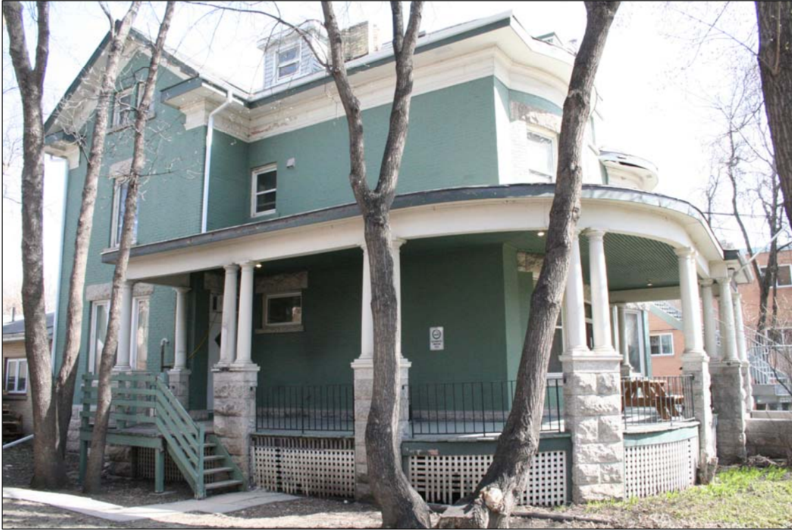
Plate 13 – 159 Mayfair Avenue, front (south) and west façades, 2008. ( M. Peterson, 2008. )
