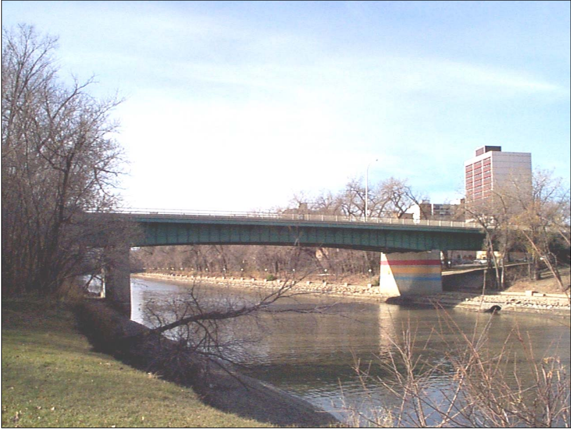
Plate 3 – Midtown Bridge, 1998. ( M. Peterson, 1998. )
