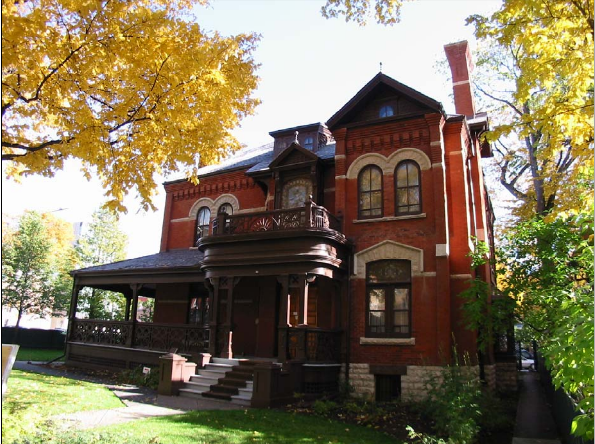
Plate 5 – Dalnavert, Sir Hugh John Macdonald House, 2003; built in 1895, architect C.H. Wheeler. ( M. Peterson, 2003. )
